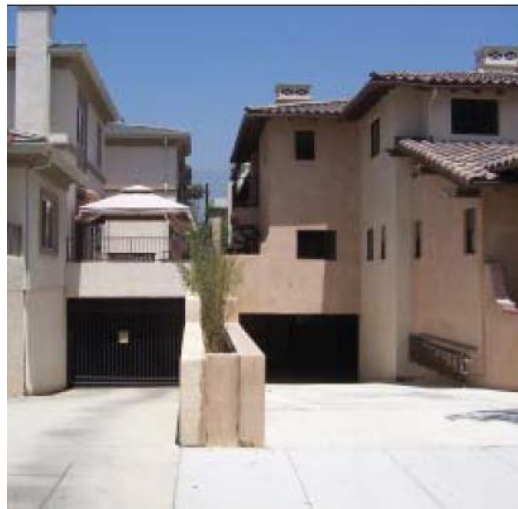
Access to Parking
