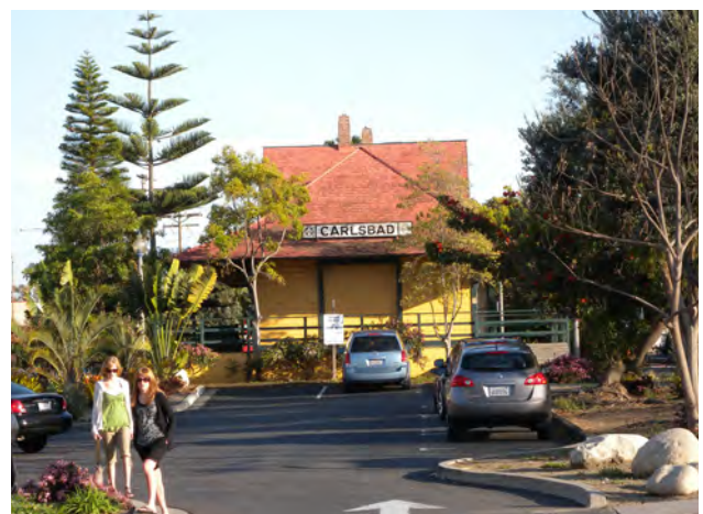
The old Santa Fe Train Depot was built in 1907 and first served as a telegraph office, post office, Wells Fargo Express office, and a general store. The top photo was taken in 1958, when the property was for sale and only a couple years before its closing. Today, it is restored as the city's Visitor's Information Center, a colorful icon in the Village (bottom).
