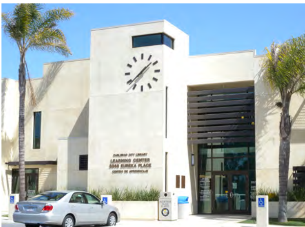
Carlsbad City Library (Dove Library) (top); Georgina Cole Library (middle); Carlsbad City Library Learning Center (bottom).
