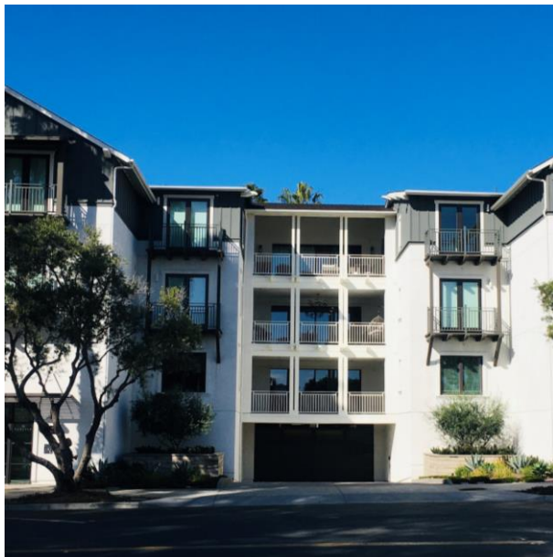
Access to Parking
