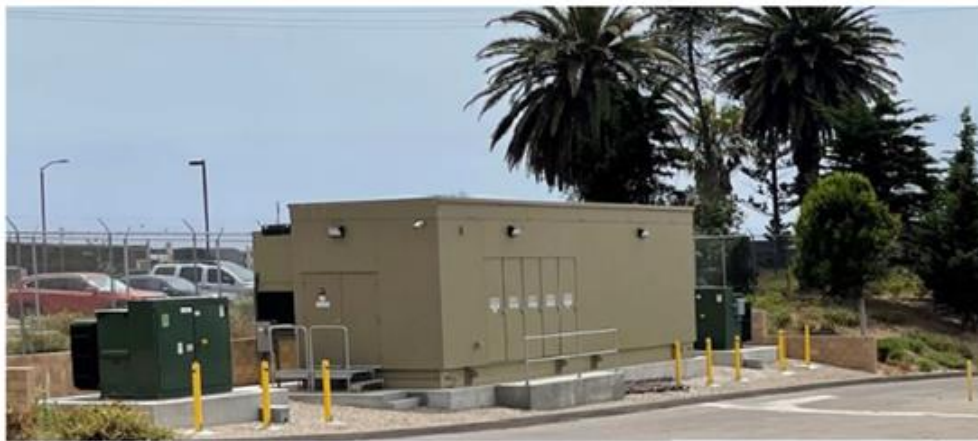
EXISTING (PHASE 1) ELECTRICAL BUILDING
