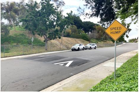
Speed cushions help reduce speeds without forcing drivers traveling at safe speeds to stop or significantly slow down.
