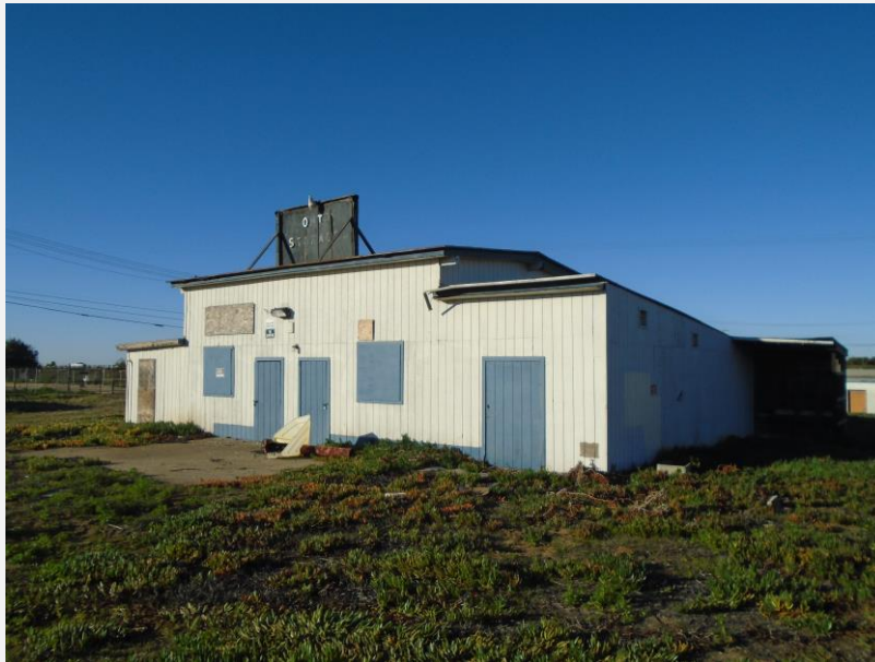
Figure 5. Office Building 1, East and north elevations, view to northwest (DSC00087).
