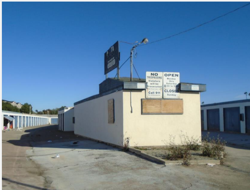
Figure 8. Storage Buildings, South elevations, view to north (DSC00199).
