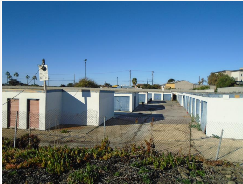
Figure 7. Storage Buildings, East and north elevations, view to west (DSC00163).
