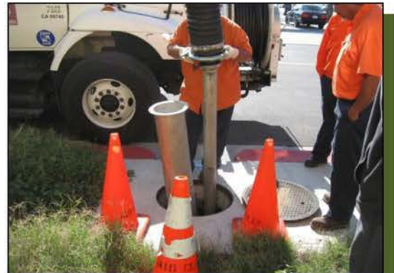
Insertion of vacuum hose into separation chamber.
