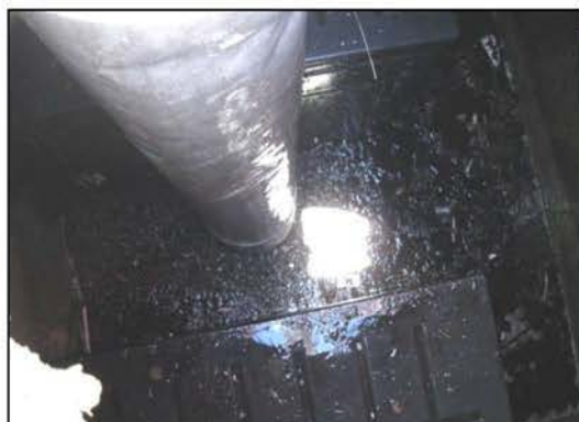
Removal of trash, sediment and debris.
