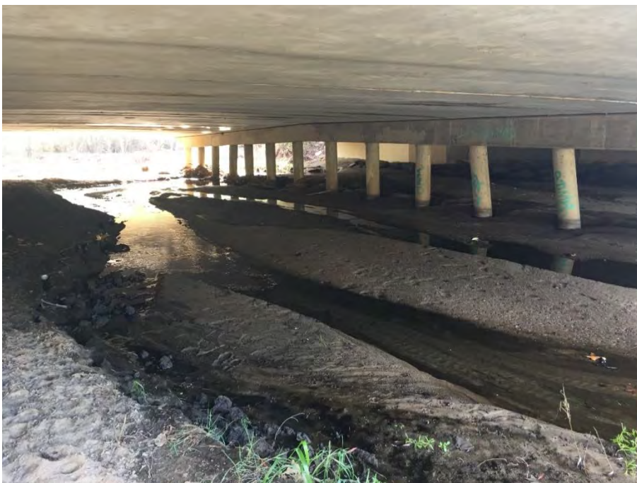
Looking south underneath the underpass at EW2-5
