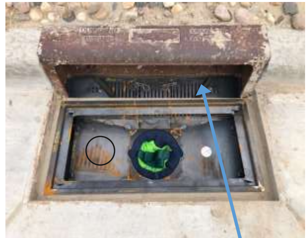
Image 3 – Installed custom made DIF-C with Mundus Bag, diverter screen, diverter wings, and sample port location
