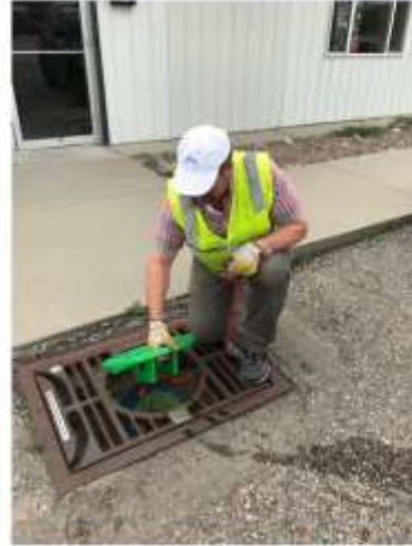
Image 6 - Opening the OGB hinged access hatch
