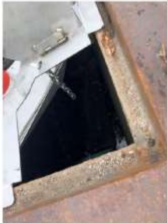
Image 11 – View of the catch basin sump through the hinged sample port located on the frame.
