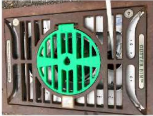
Image 9 – Sample port being pivoted with grate in place to view bottom of catch basin
