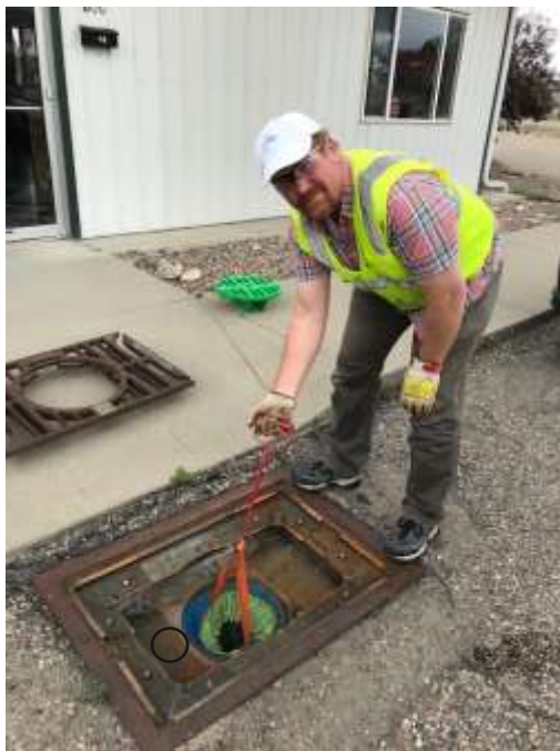
Image 8 - Demonstrating Mundus Bag removal for a DIF with grate removed
