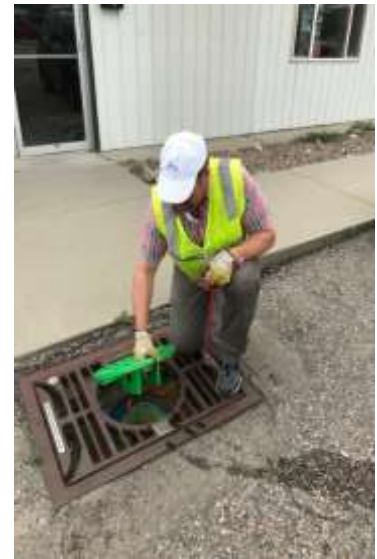
Image 11 - Demonstrating the closing of the OGB access hatch
