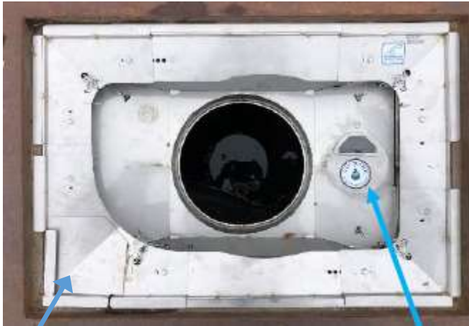
Image 2 – Adjustable DIF with closed sample port and without a Mundus Bag
