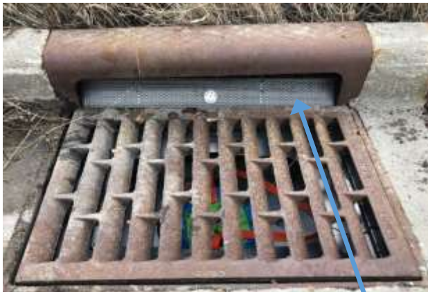
Image 4 – Installed DIF-C below the existing storm grate cover and an inlet screen in curb inlet opening
