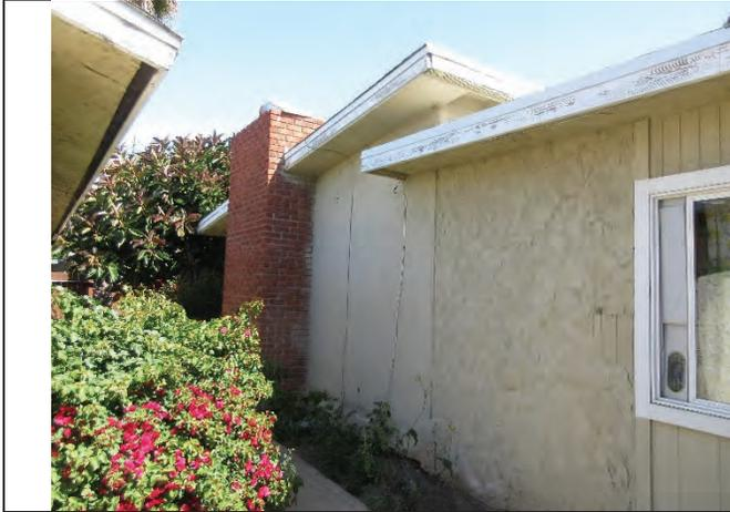
**Image 1.** Textured stucco over wood siding beside window, with smooth stucco adjacent to chimney, south end of west facade.
