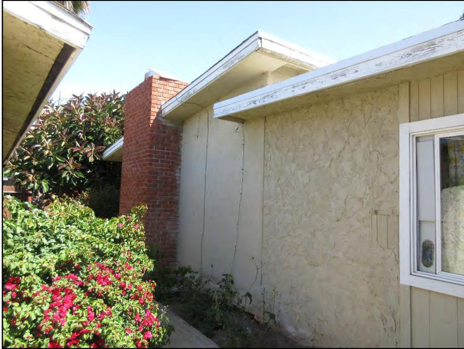
Figure 19. Textured stucco over wood siding beside window, with smooth stucco adjacent to chimney, view to north-northwest.
