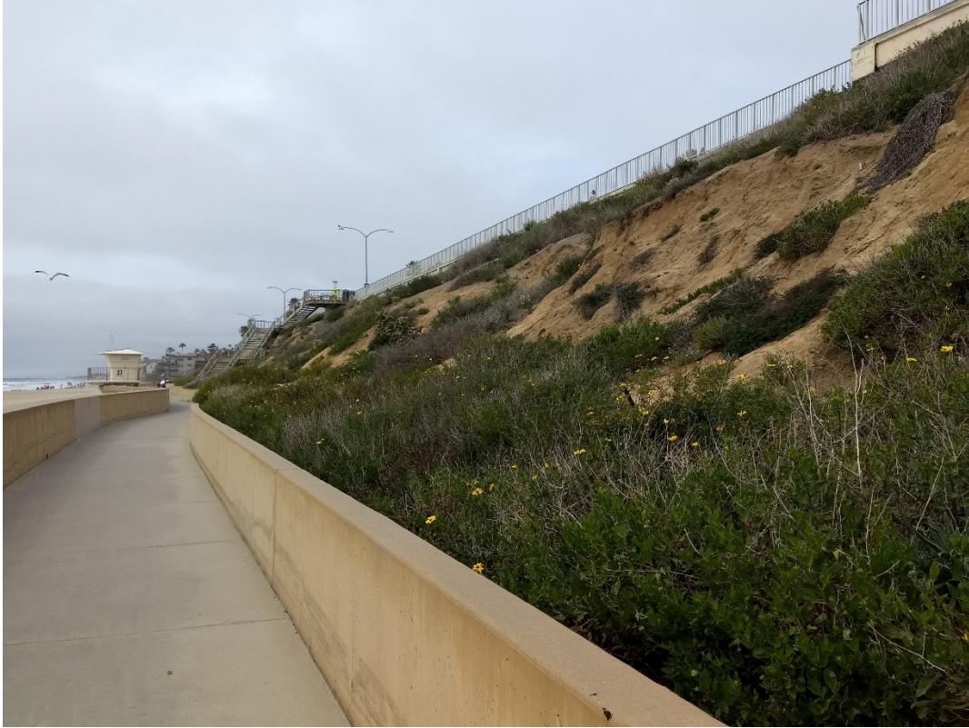
Photograph #5: Bluff near North end looking Northwest
