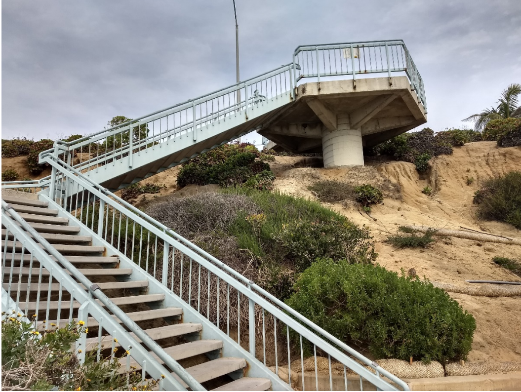
Photograph #3: Stairway Opposite Hemlock Avenue looking East
