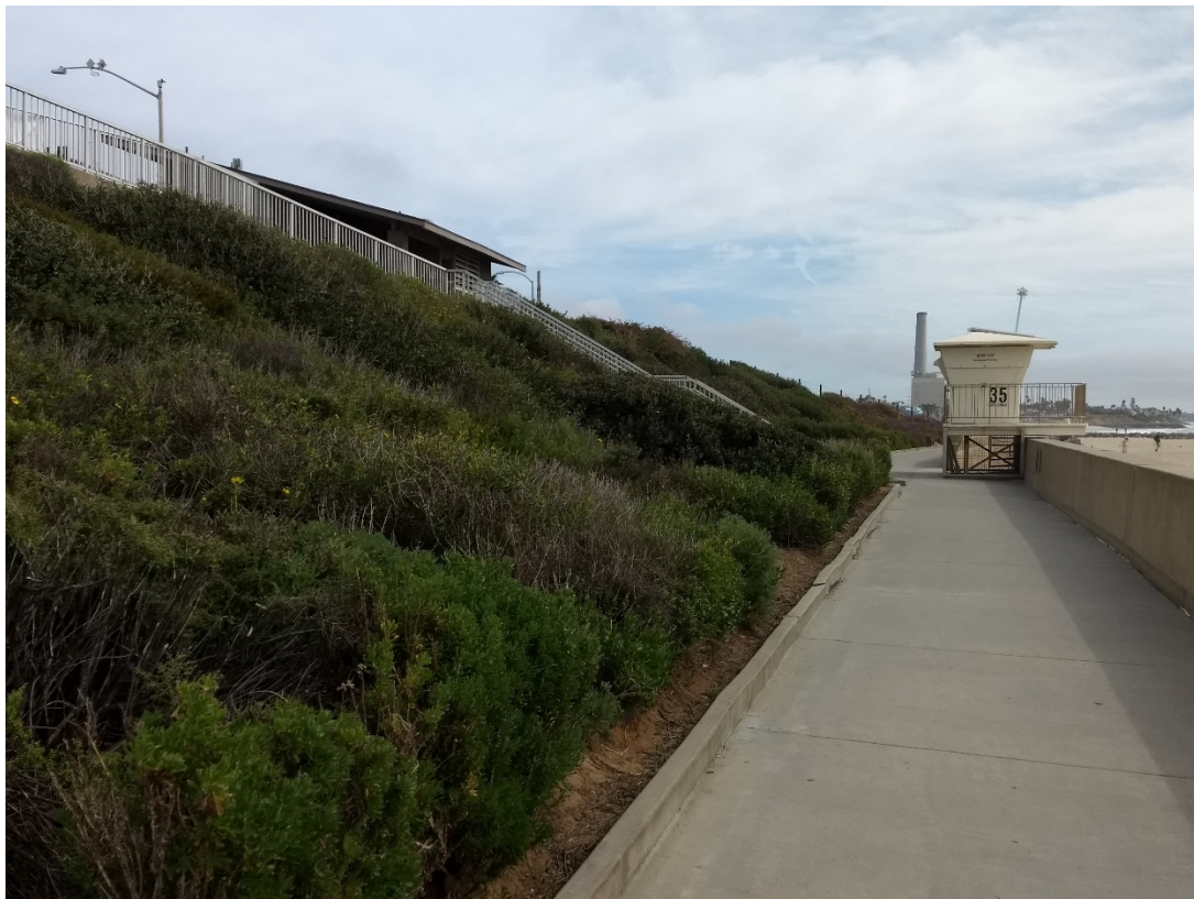
Photograph #2: Near South end of the Project looking Southeast
