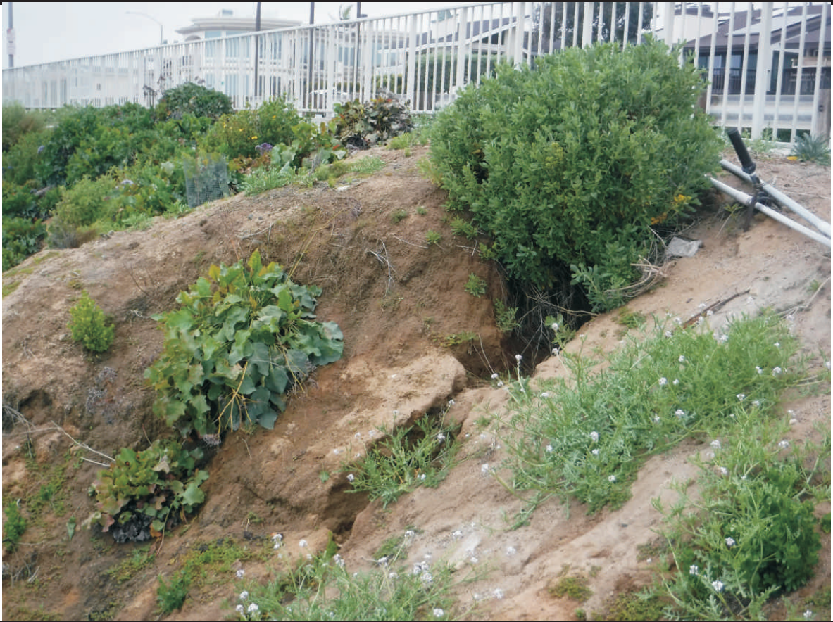
GULLY AND WET SOILS (Due to irrigation leak?)
