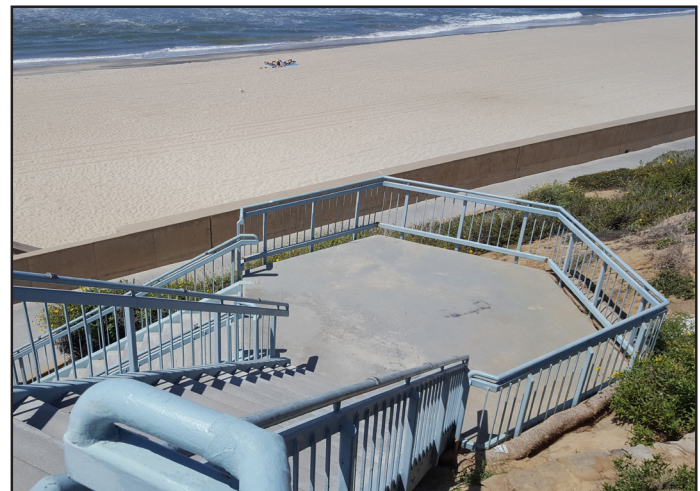
Photograph 6 Access stairs between upper sidewalk and lower walkway, looking down
