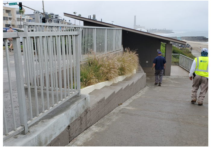
Photograph 2 Looking south down the ramp at the south end restroom
