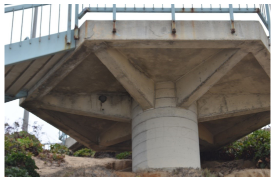
Figure 10: Beach Access Stairway 48-inch Diameter Support Piles to Remain
