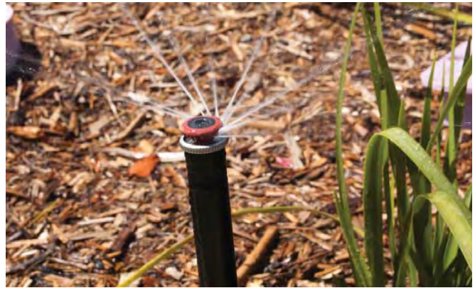
Rotator nozzles throw streams of water with larger water droplets which helps to prevent misting and runoff, but each nozzle still needs to be checked periodically to ensure it is running correctly.
