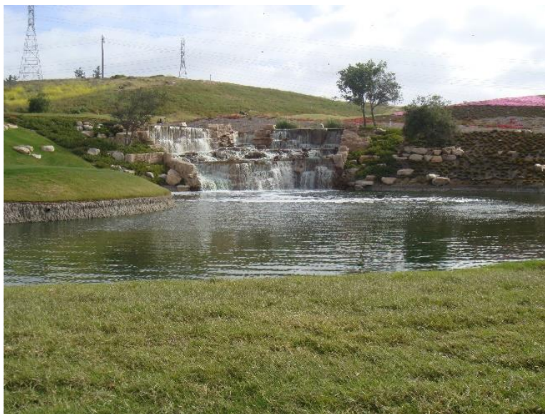
Recycled water use at golf course in CMWD's service area
