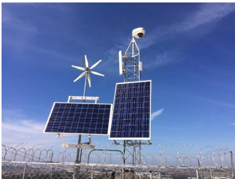
Solar and wind power used at CMWD's off-grid Santa Fe II facility
