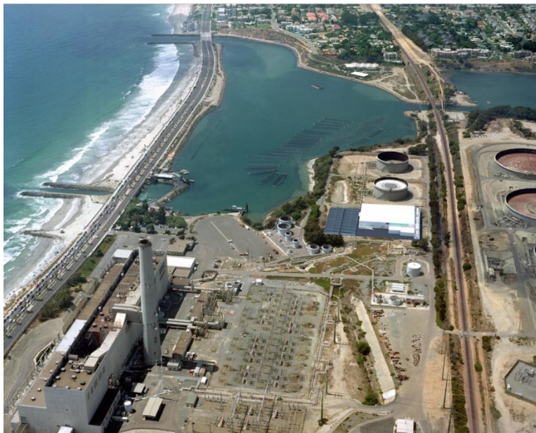
Claude "Bud" Lewis Carlsbad Desalination Plant is located adjacent to the Agua Hedionda Lagoon
