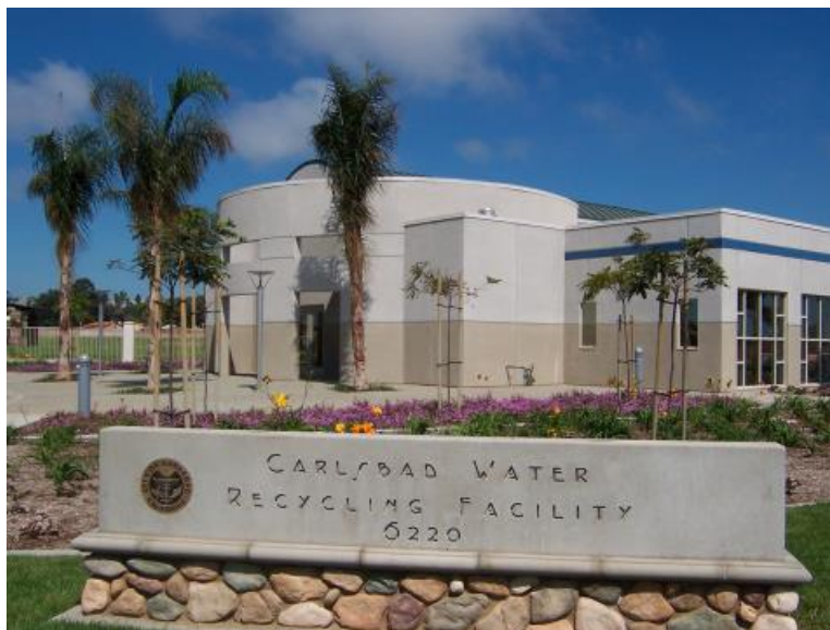
Carlsbad Recycled Water Facility (Carlsbad WRF)
