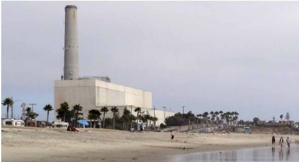
Former Encina Power Station along Carlsbad Blvd.
