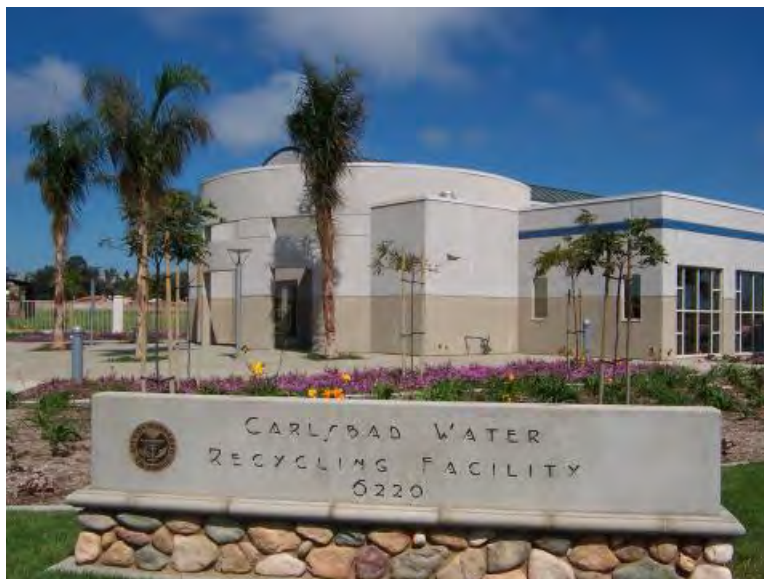
Carlsbad Recycled Water Facility (Carlsbad WRF)
