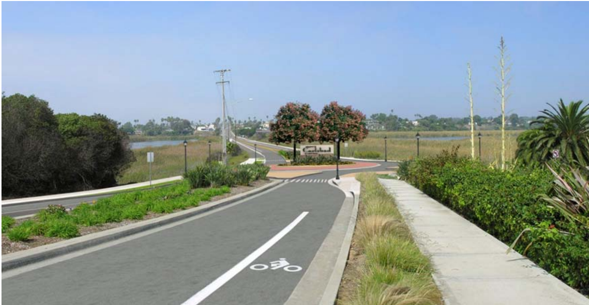
The State Street/Carlsbad Boulevard Roundabout is one of the innovative roadway improvements being implemented by the City.
