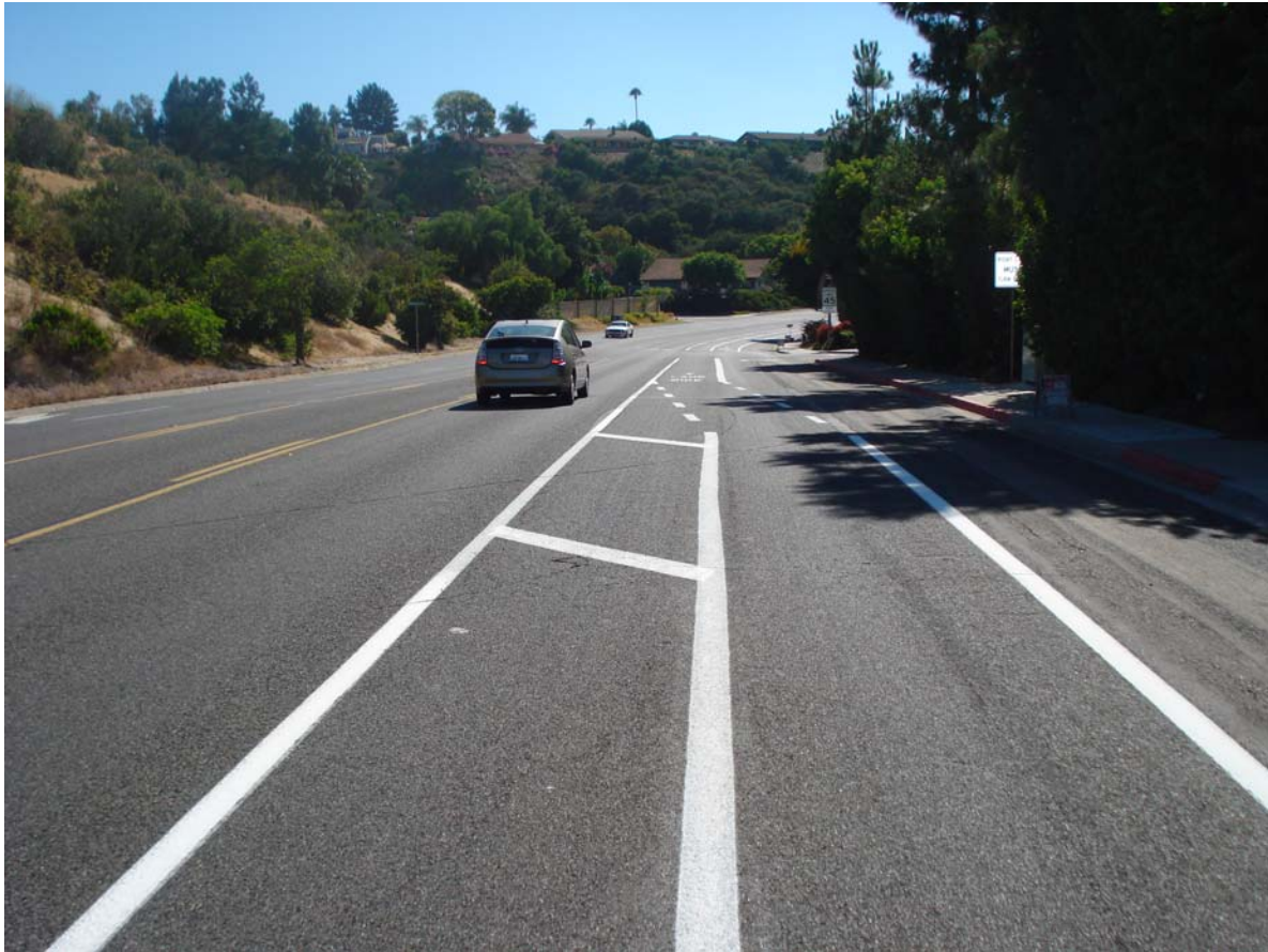
The La Costa Avenue road diet has slowed traffic without affecting emergency response times.
