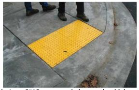
prior to 2002. On streets that have been constructed since 2002, truncated domes should be installed.
