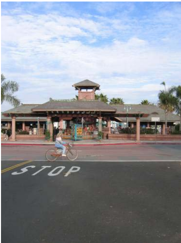
Carlsbad Village Station is accessible to bicyclists and features bicycle racks and lockers
