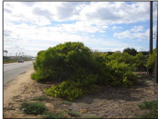
A Class I path could be located on the shoulder between the southbound lanes and the campground.
