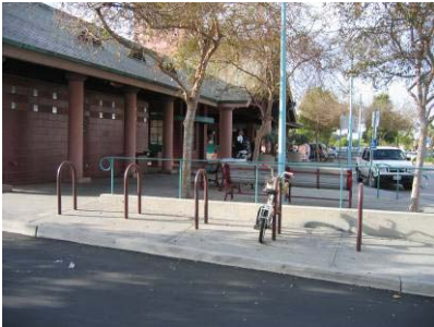
Carlsbad Village Station features inverted U-style racks
