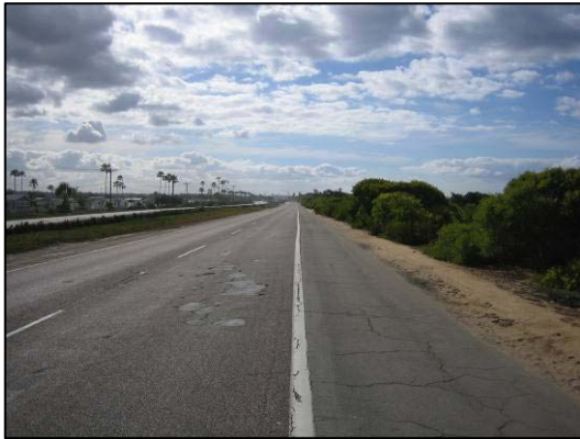
Coast Highway south of Palomar Airport Road.
