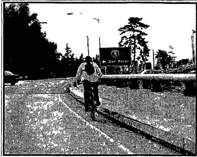
Roadway widths tend to decrease at bridge crossings and high curbs make marginal lanes even narrower This bridge over I-5 was recently rebuilt and upgraded, but similar bikeway situations still exist on other bridges in Carlsbad
