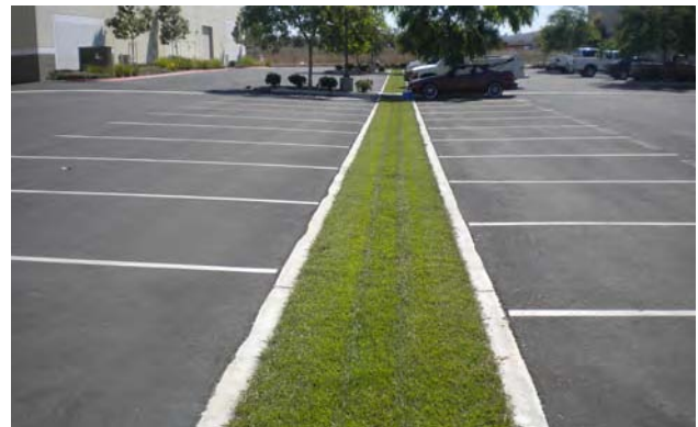
Green design features include parking landscape treatments such as this gradual pavement grade draining through an “O” curbface directly to a vegetated swale. The turf-block under the planted grass is a concrete structure with openings to allow vegetation to grow and for drainage filtration of hydrocarbons and other pollutants to be absorbed and treated with the organic plant material. The turfblock system also allows for traffic and vehicle access without failure or damage to the vegetation.
