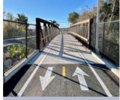
Inland Rail Trail at the Buena Creek bridge (Source: SANDAG)
