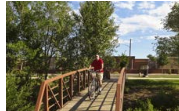
Santa Fe River Trail Bridge
