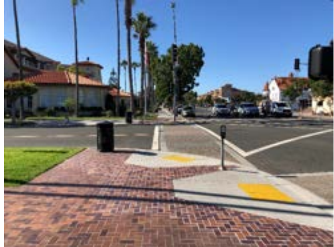
An example of a high-quality pedestrian intersection.
