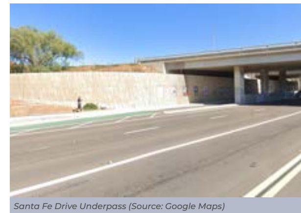
Santa Fe Drive Underpass (Source: Google Maps)
