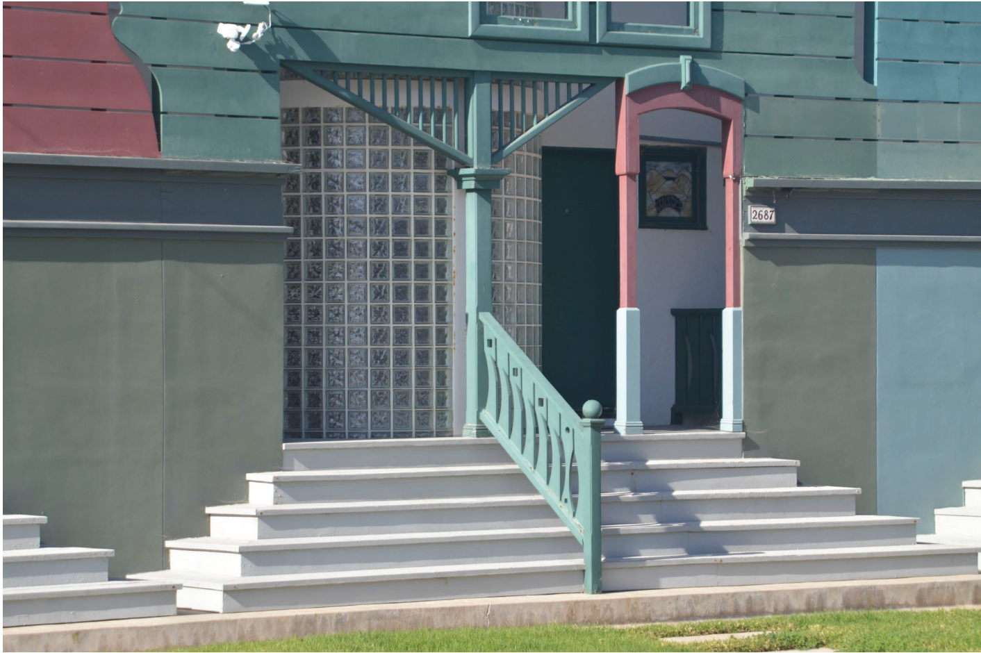
At Victor Condo, the fascia boards, horizontal siding, the steps, cut out railings, and spindle details come directly from the Magee Park buildings
