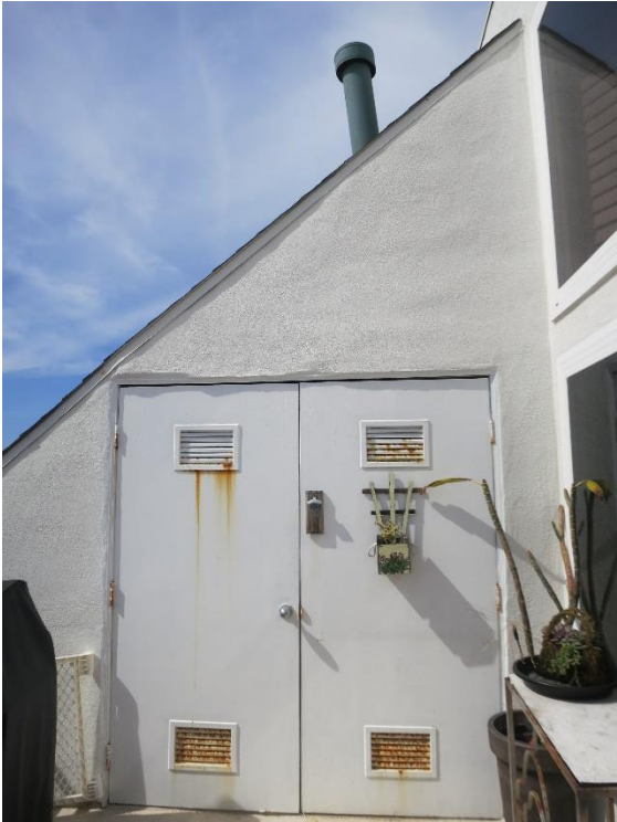
Figure 26. Detail of storage doors and shed roof, view to the north.
