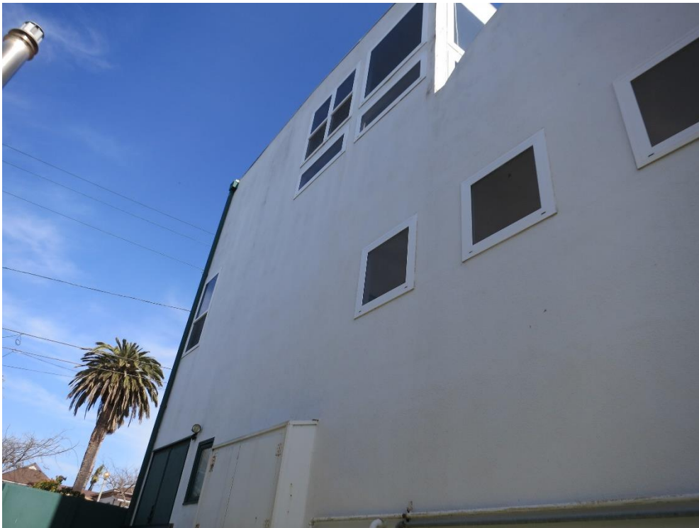
Figure 30. View of north façade of the property, view to the southeast
