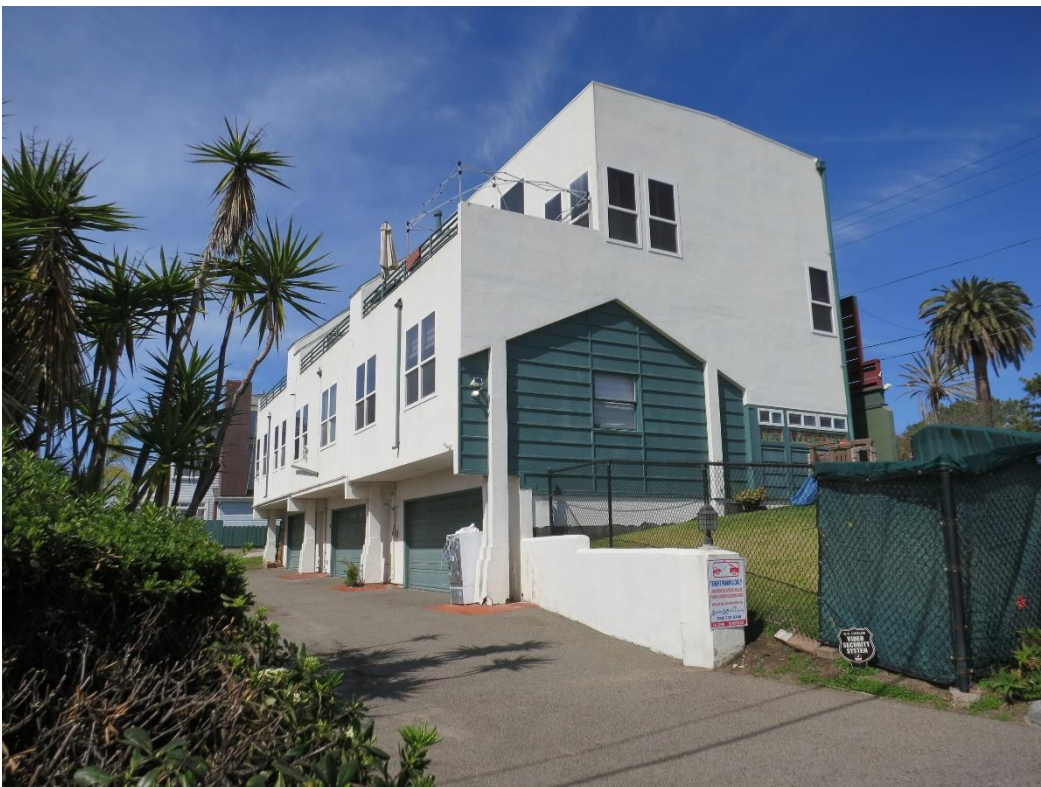
Figure 11. View of south façade of property, looking northeast
