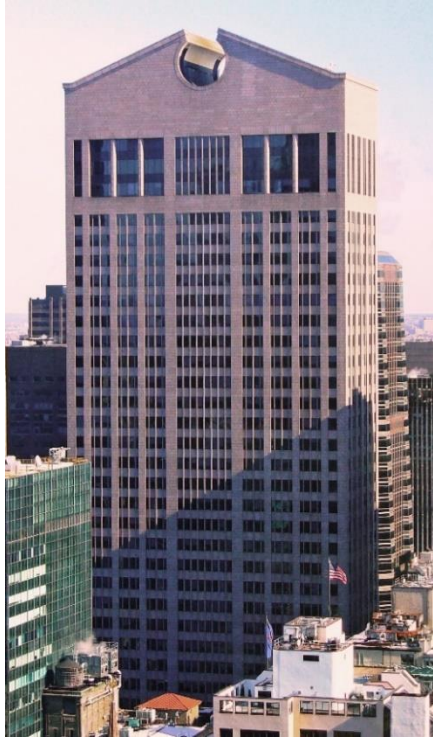
Figure 5. Johnson's AT&T building. Photo by David Shankbone.
