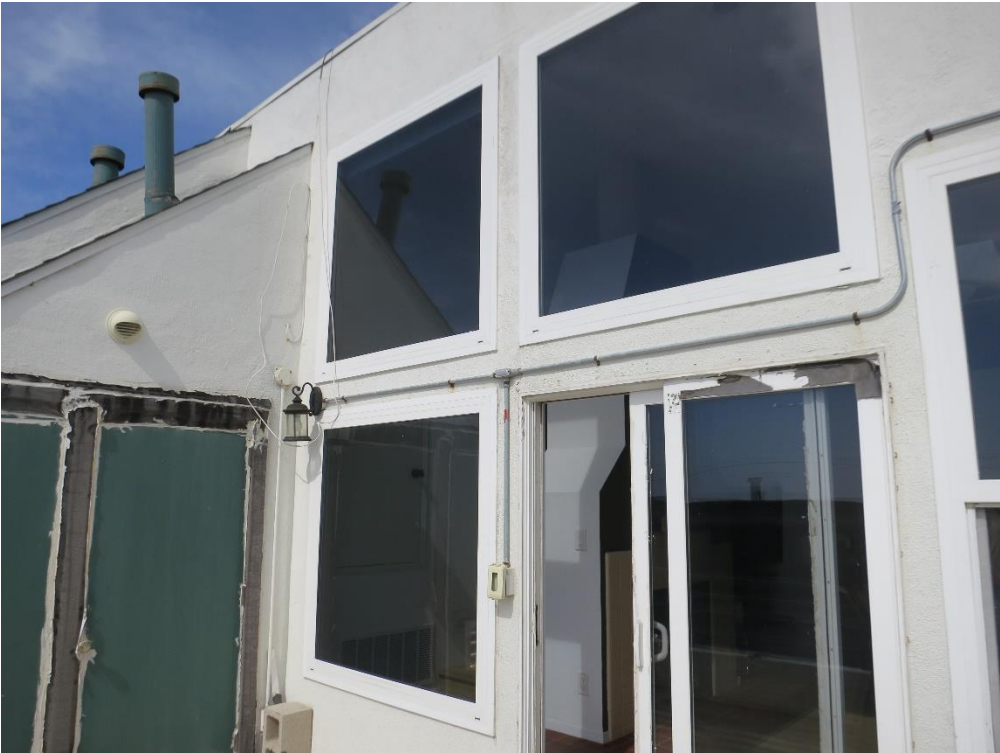
Figure 27. Detail of fenestration on south facade, view to northeast
