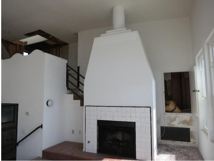
Figure 41. Detail of fireplace in 2685 Garfield St., view looking south
