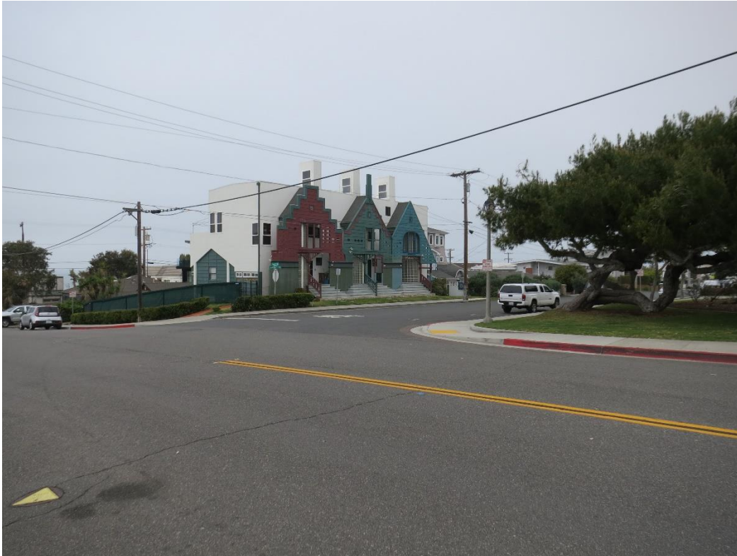
Figure 10. Overview of Victor Condo, view to the northwest
