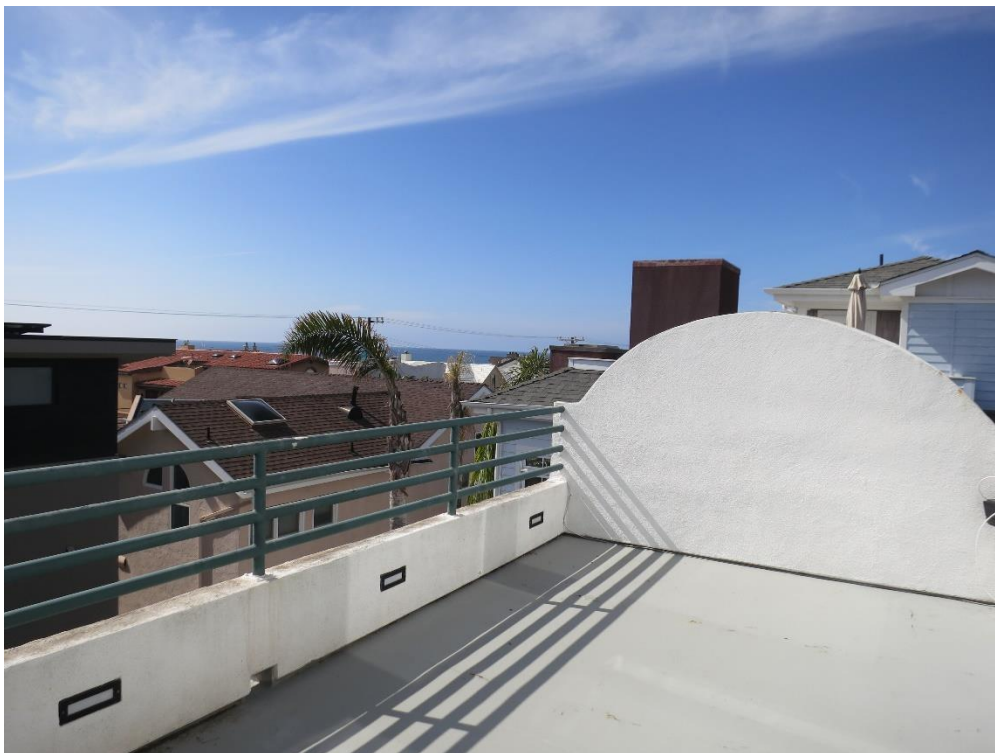
Figure 29. Detail of rounded balustrade of 2689 Garfield St., view to northwest
