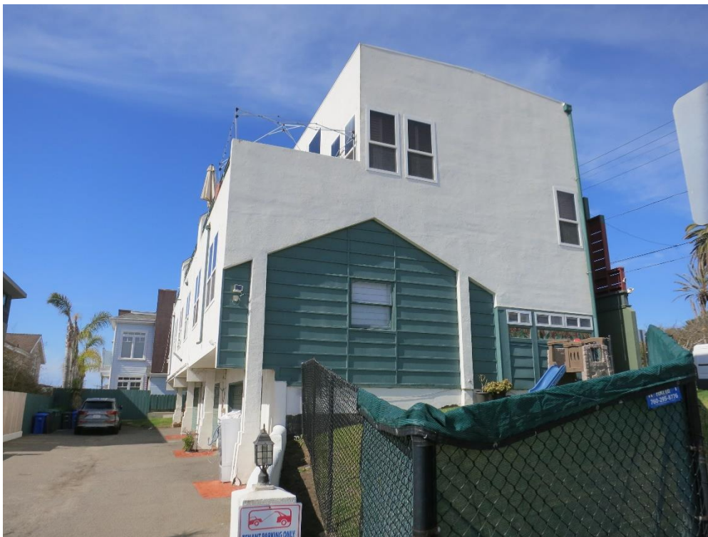
Figure 23. View of south façade of property, view to north
