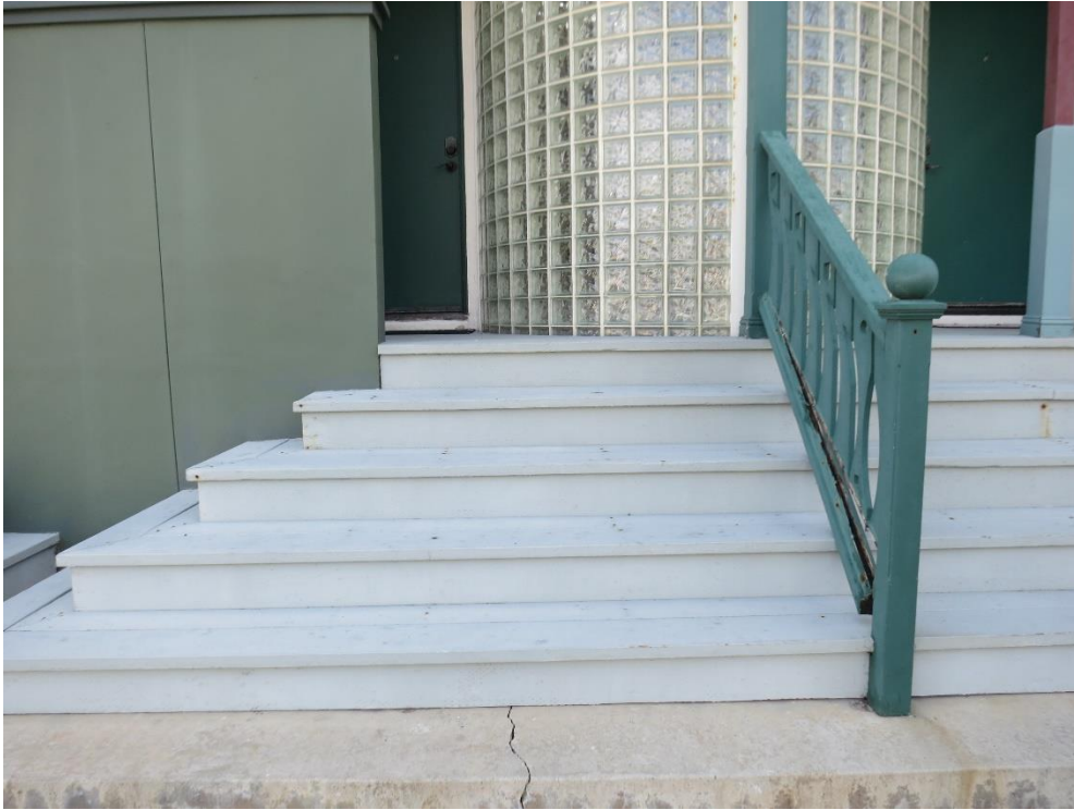
Figure 18. Detail of steps of 2687 Garfield St., view to the west
