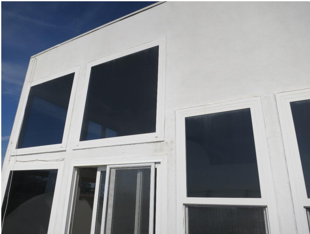
Figure 28. Detail of fenestration on 2689 Garfield St., view to the east
