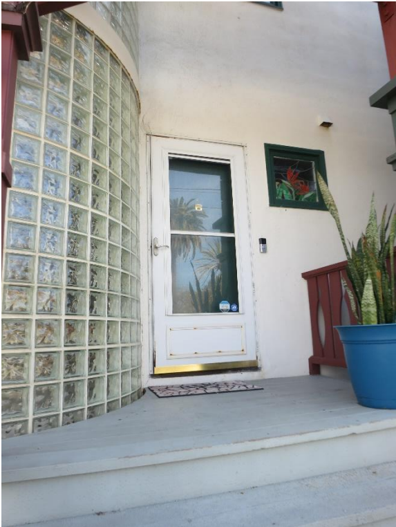
Figure 21. Detail of door and entrance of 2689 Garfield Street, view to northwest
