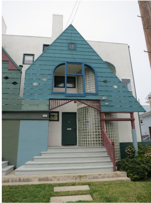
Figure 14. Detail of front façade of 2685 Garfield St., view to the west
