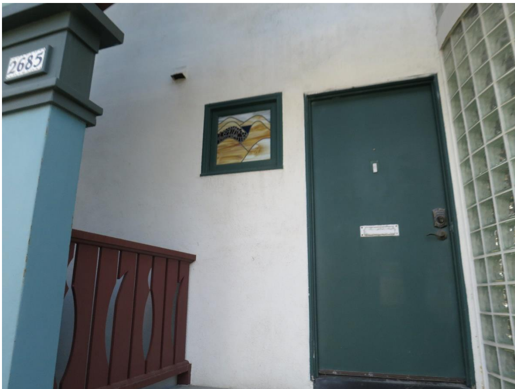
Figure 15. Detail of door and balustrade of 2685 Garfield St., view to west
