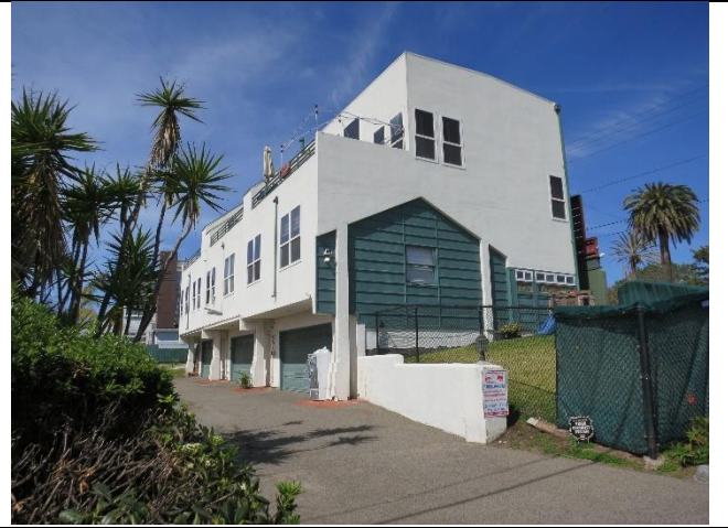
Image 2. South façade looking north.
