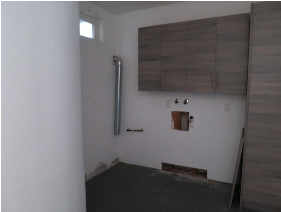
Figure 32. View of laundry area on ground floor of 2687 Garfield St.
