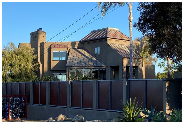
Figure 51. Another Postmodern house in Carlsbad built in 1984.
