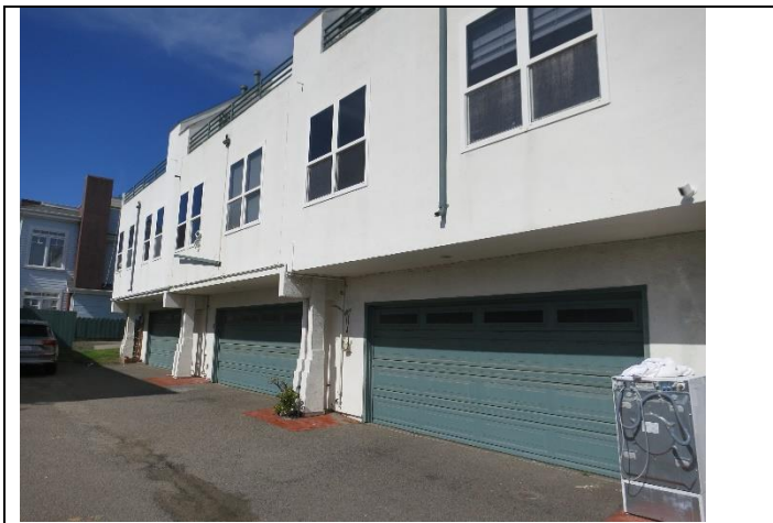
Image 3. View of west façade of Victor Condo, looking NE.
