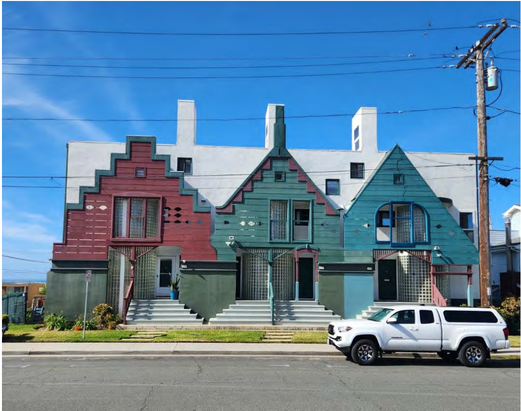
Facade of 2685/2687/2689 Garfield Street Building in Carlsbad. View to SW. March 7, 2023.
