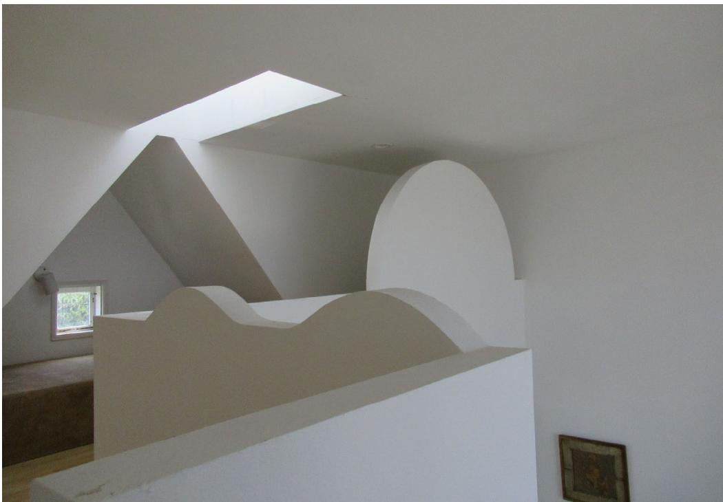
Photo 34: Shaped parapet walls at Mezzanine B.
