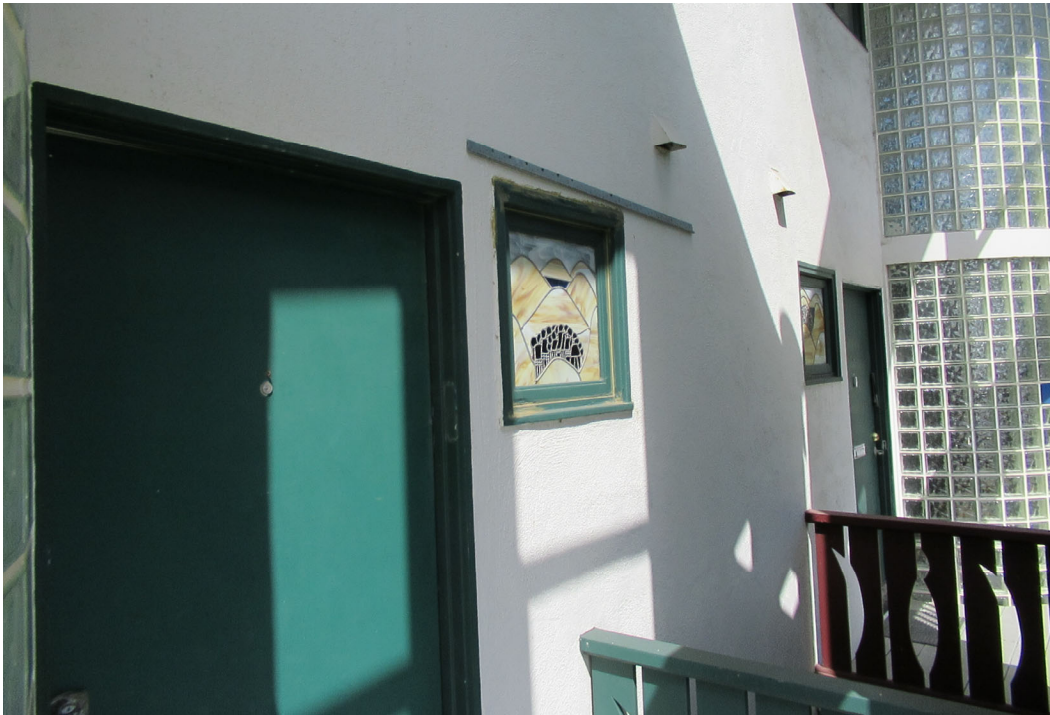
Photo 11: Two original stained-glass windows of the east façade.
