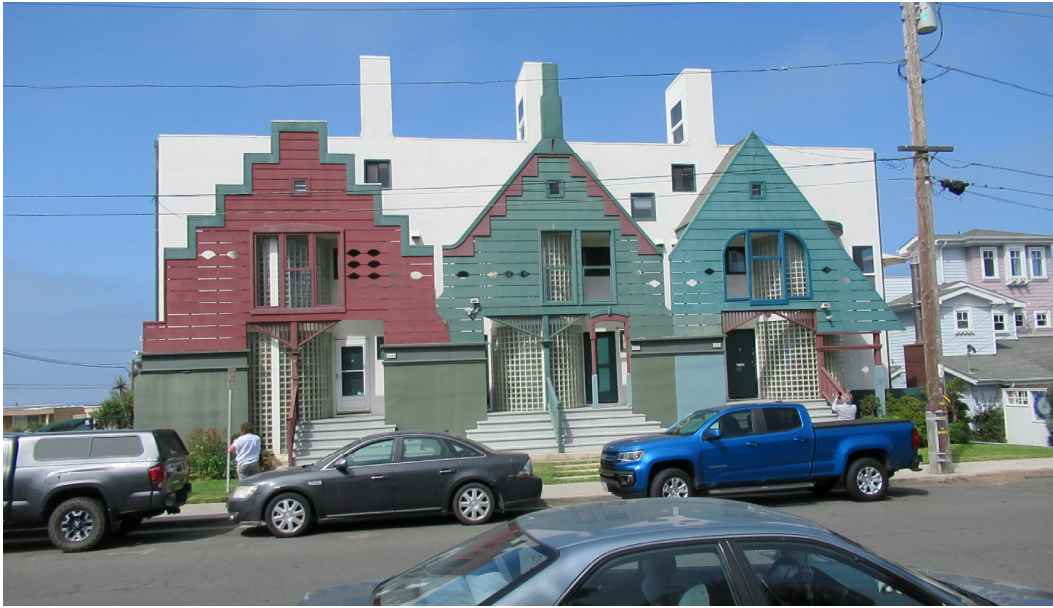
Photo 1: The Victor Condo Building looking west at the primary (east) façade showing the building's distinctive false front façade.
