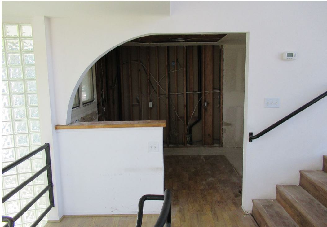
Photo 17: Original kitchen entrance in Unit 2685. Looking south from the Dining Room.
