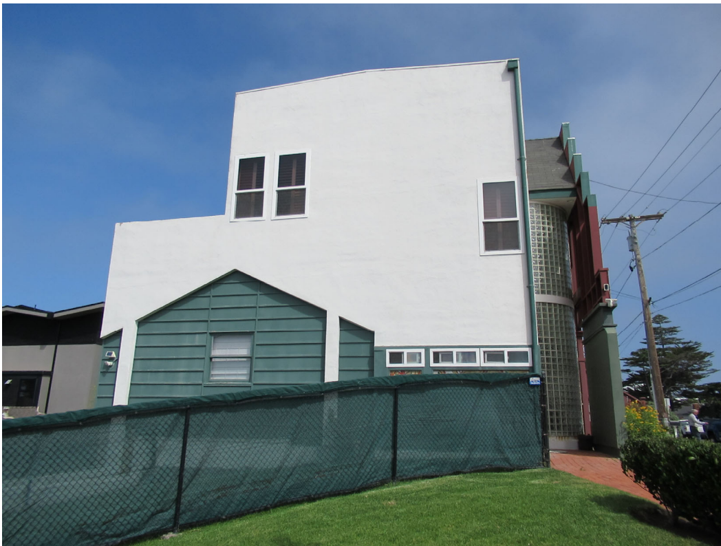
Photo 2: The south façade looking north. There is one original wood double-hung window. The other windows have been replaced.
