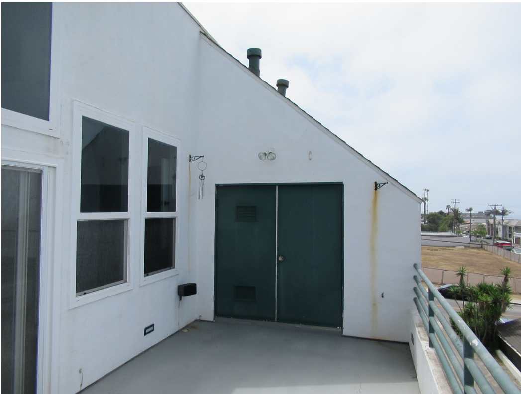
Photo 22: Balcony C at Unit 2685 looking south at the mechanical closet.
