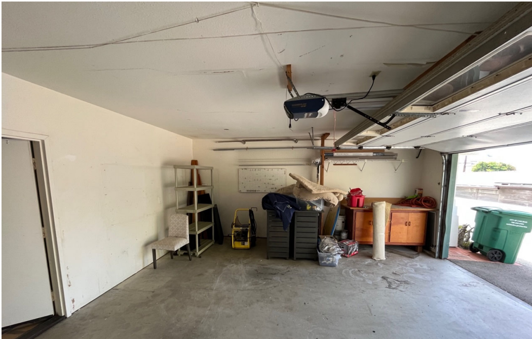
Photo 25: Garage B in Unit 2687 looking south.
