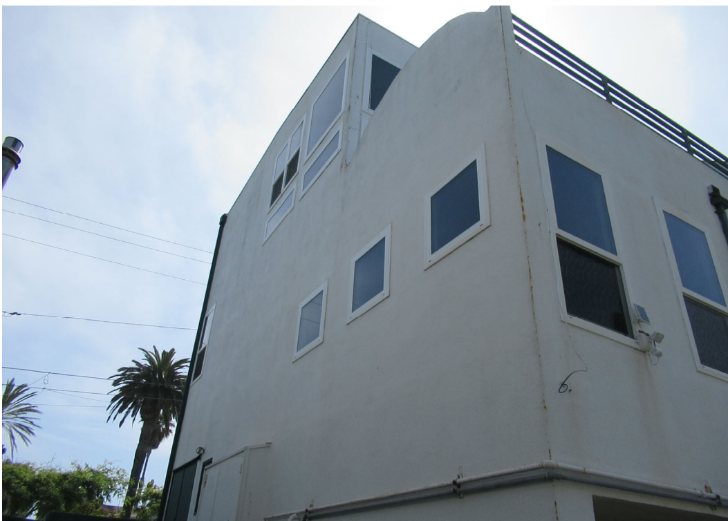
Photo 4: the north façade. All of the windows have been replaced.
