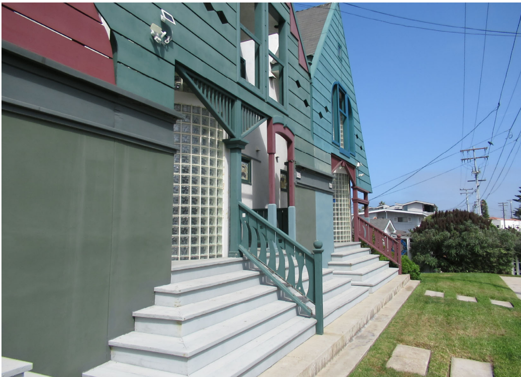
Photo 6: Front façade showing the existing wood steps, wood rails, and other decorative elements.
