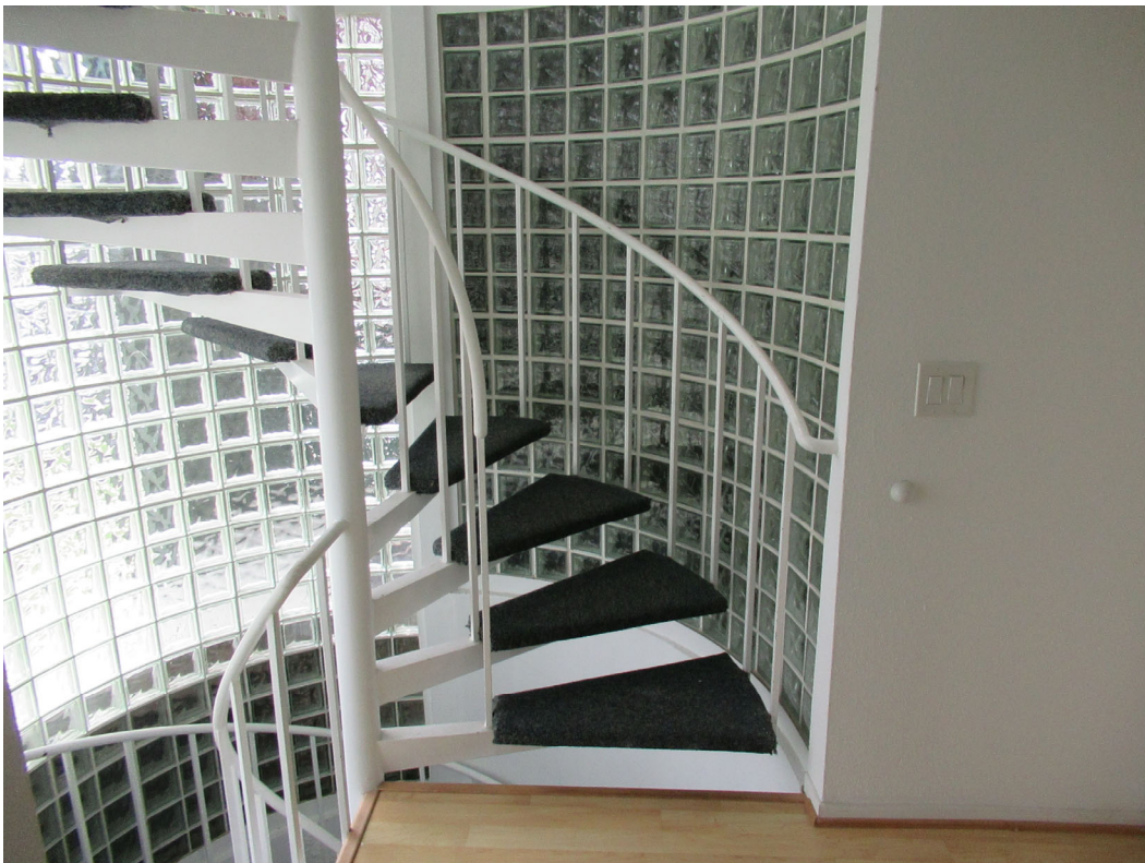
Photo 26: Entry B looking east at the original spiral stairs.
