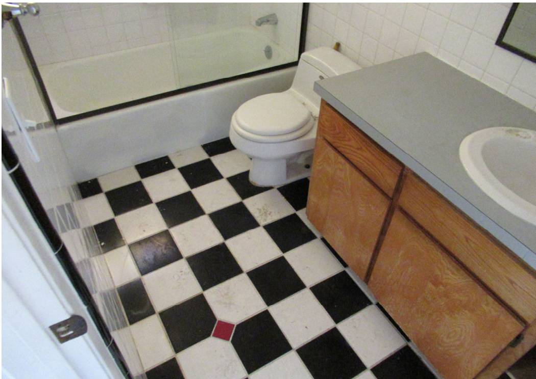
Photo 14: Original finishes in Bathroom 2C.
