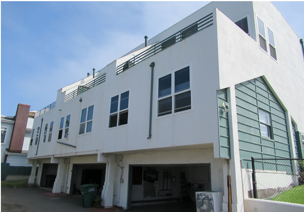
Photo 3: The rear (west) façade looking northeast. All of the windows and exterior doors on the west façade have been replaced.
