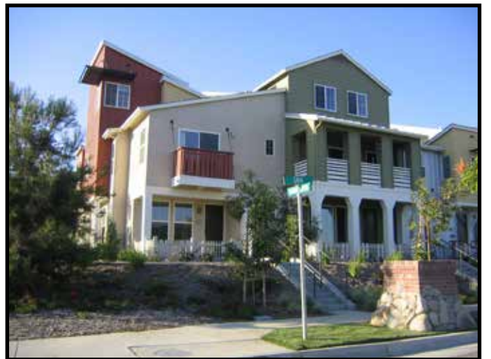
Articulated roof forms
