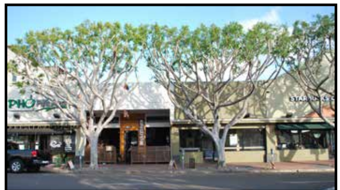
Continuous, pedestrian-oriented street frontage
