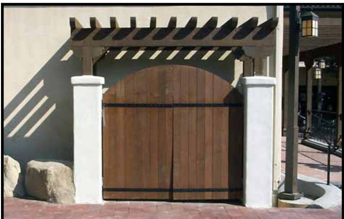
Screened service area
