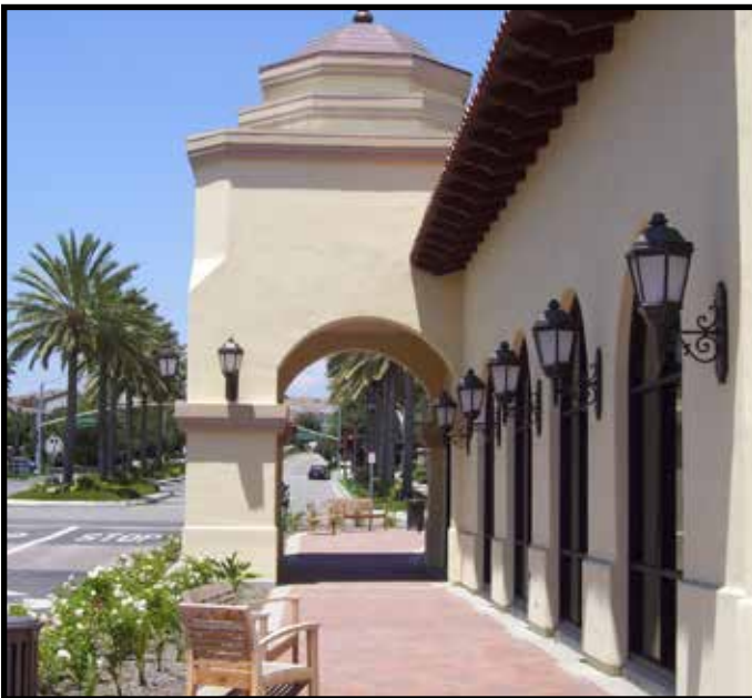
Vertical building focal element
