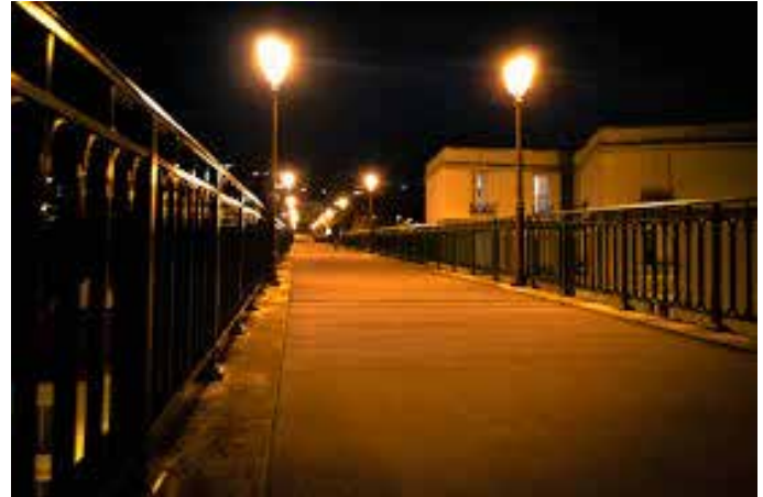
Night street lighting
