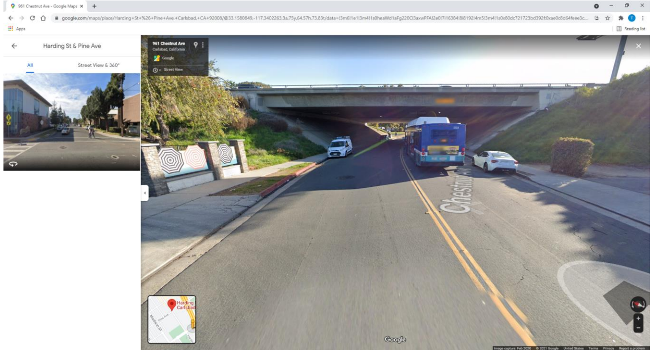
Entering from Harding Street headed east (Prior to construction)
