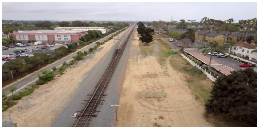
NCTD Rail Corridor – Potential to add more parking as a shared resource
