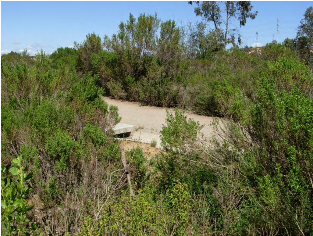
M11-2, west side looking northeast.
