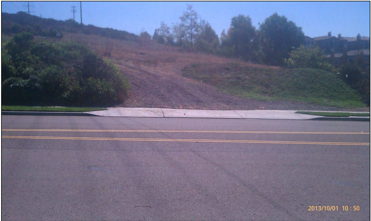
M8-2, at-grade crossing west side facing east, October 2013.
