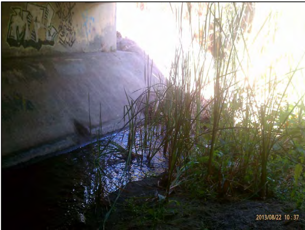
EW1-6, looking north from west entrance, August 2013.
