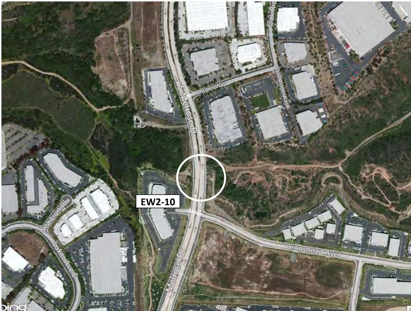
EW2-10. High Priority. Does not appear to be any fencing.
