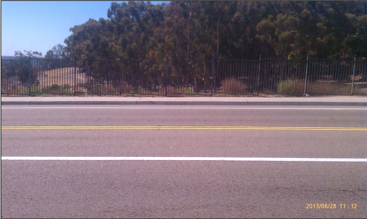
M1-1, north side facing south; note fencing, August 2013.
