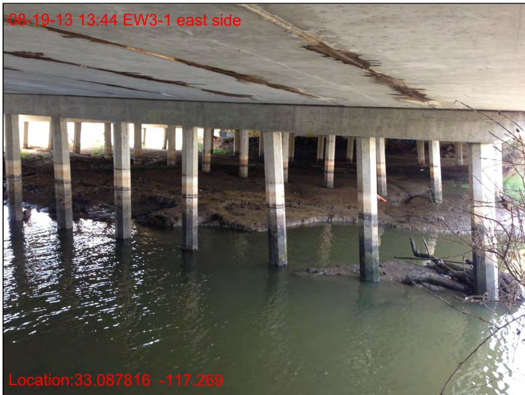
EW3-1, looking east at 20 meters from west entrance, August 2013.
