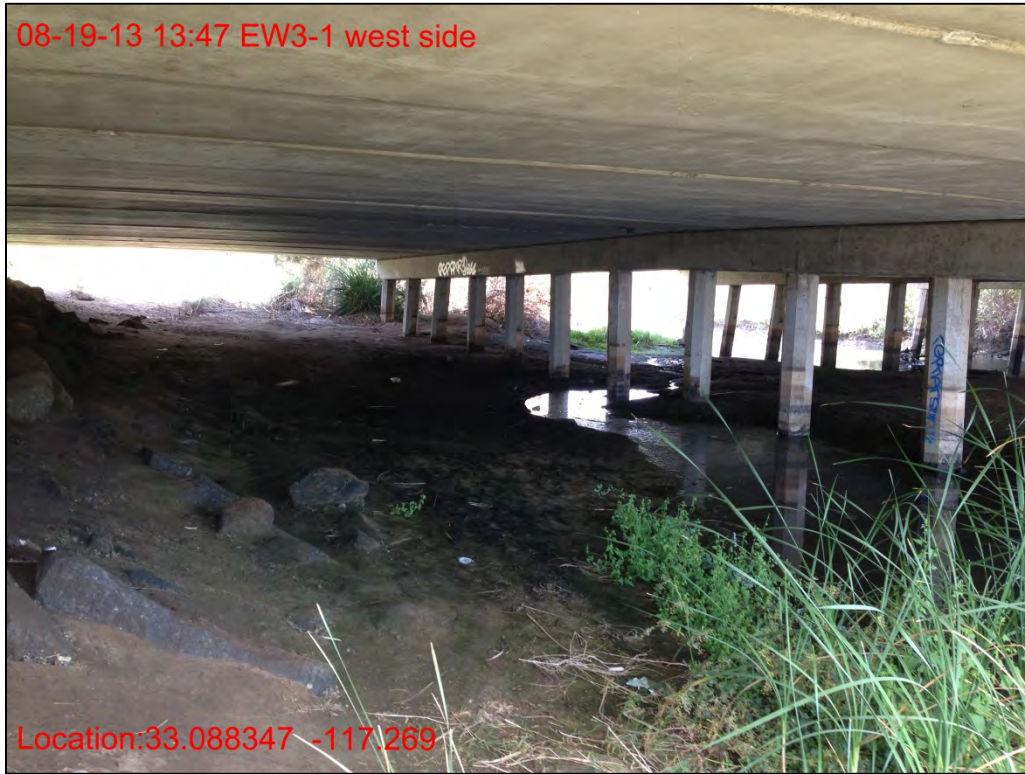
EW3-1, looking east from west entrance, August 2013.
