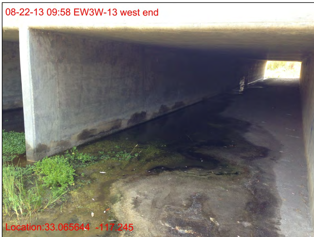
EW3-13, looking east from west entrance, August 2013.
