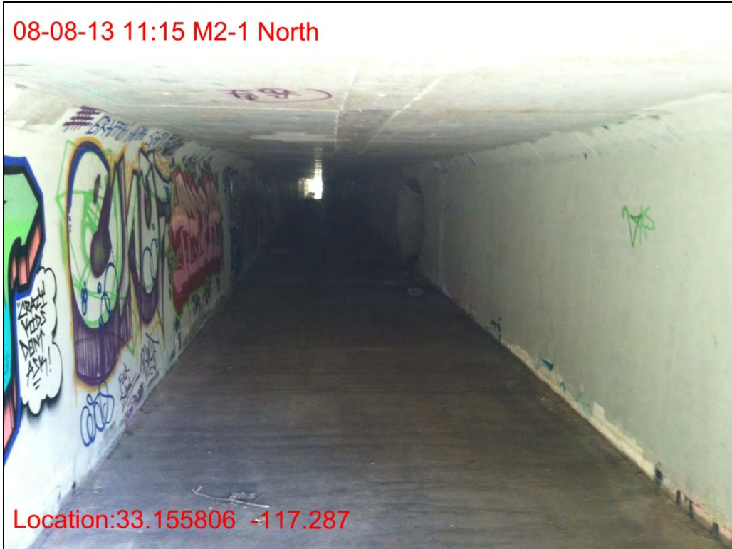
M2-1, north end facing south into undercrossing, August 2013.
