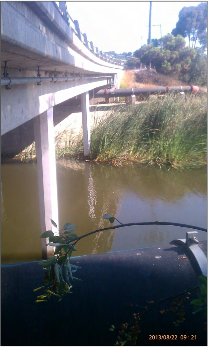
EW1-3, looking south along east entrance, August 2013
