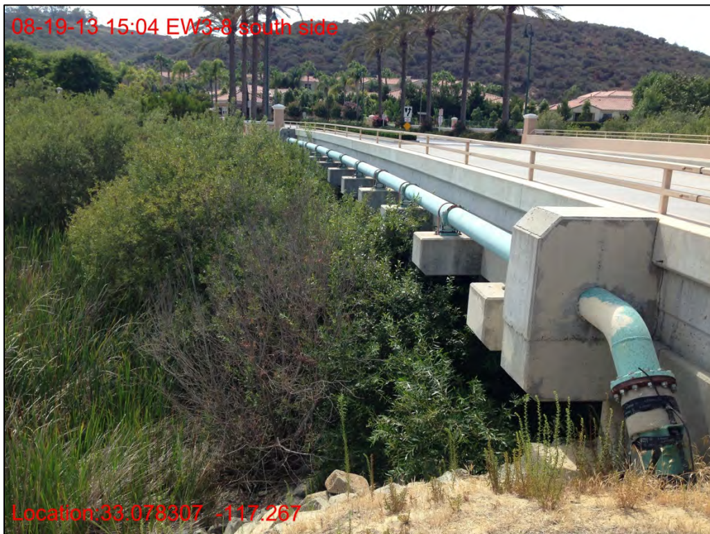
EW3-8, looking west from south end, August 2013.
