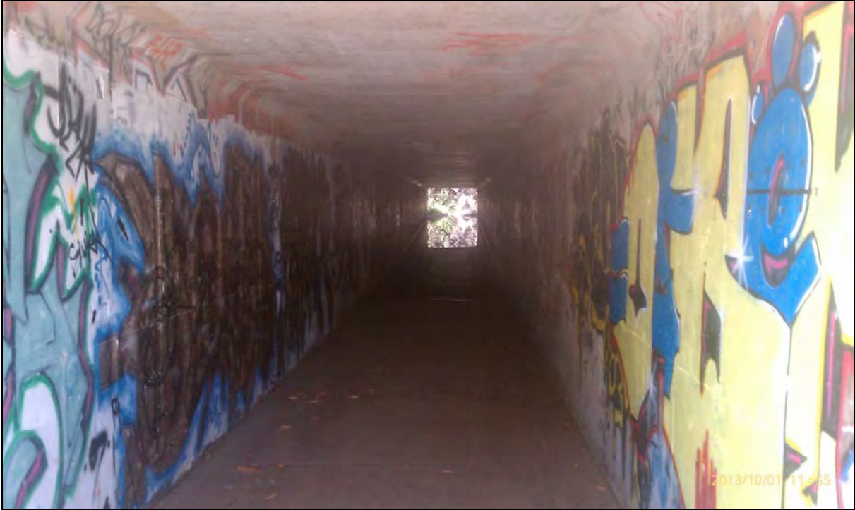
M6-2 east entrance looking west, October 2013.
