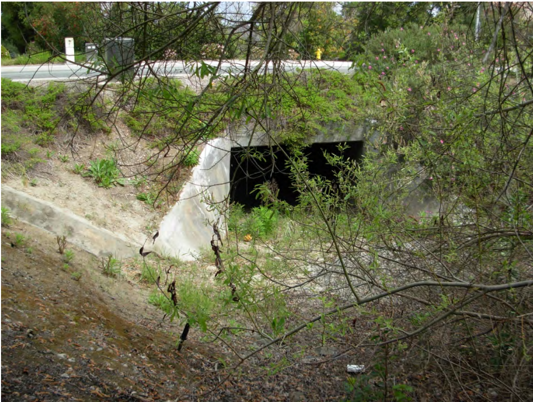
M5-1, looking north at 20 meters from south entrance.
