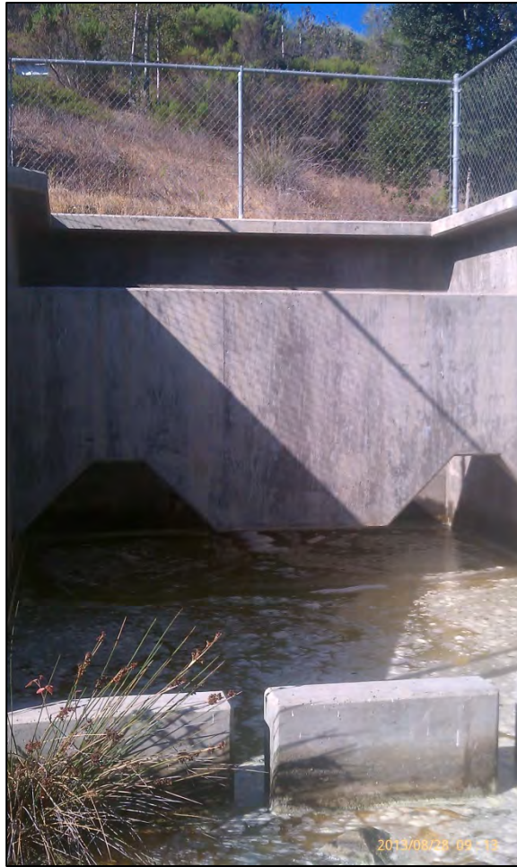
M7-1, north side showing constraints, August 2013.
