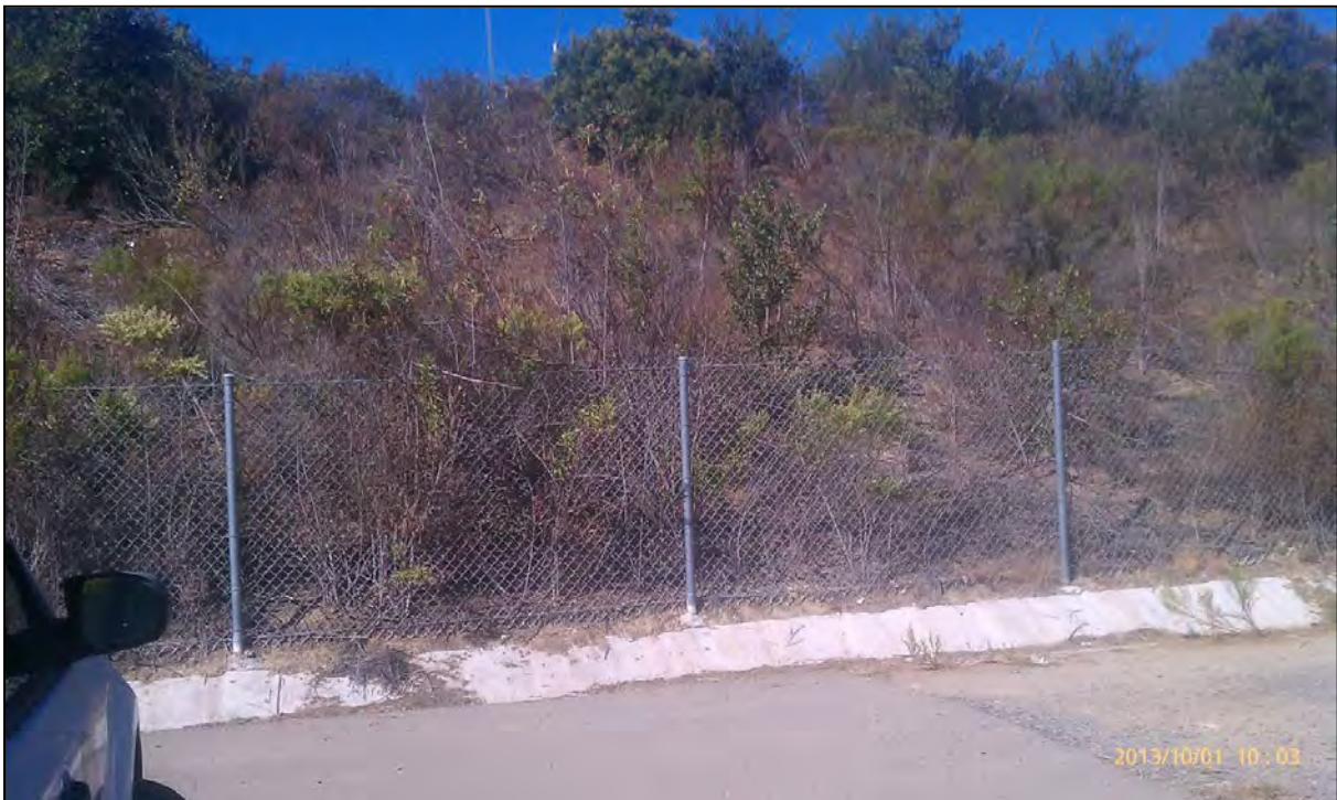
CC3-3a, east side looking west from access road, showing fencing, October 2013.
