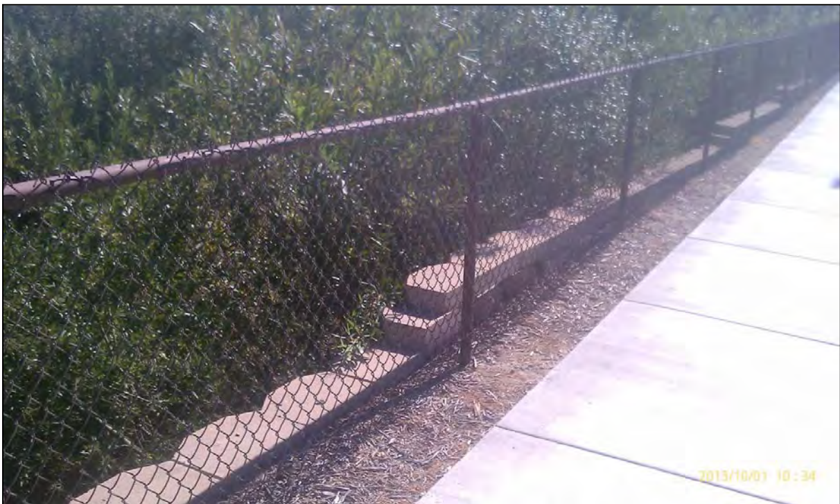
CC3-2 west side, showing fencing, October 2013.
