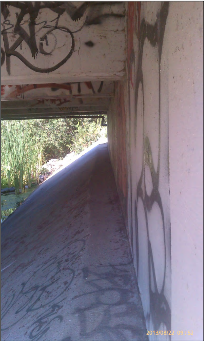
EW1-5, looking east on south side, August 2013
