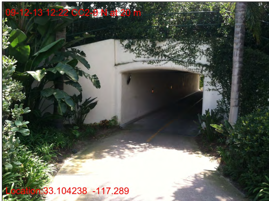
CC2-9, north side at 20 m out, September 2013.
