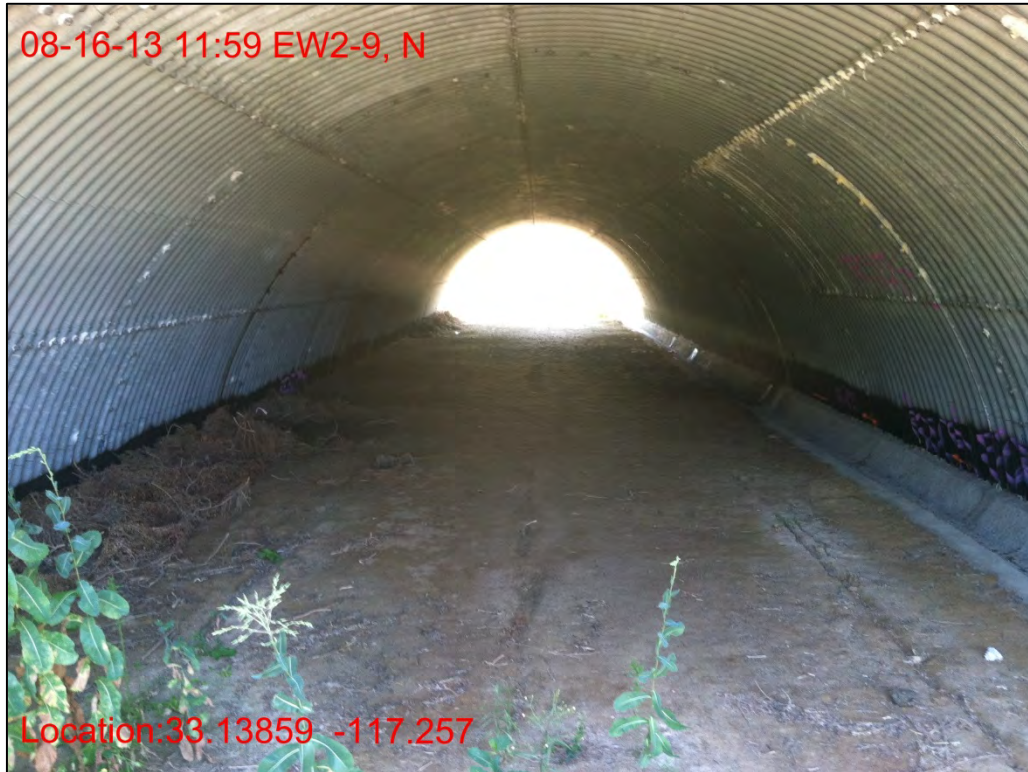
EW2-9, looking south from north entrance, August 2013.
