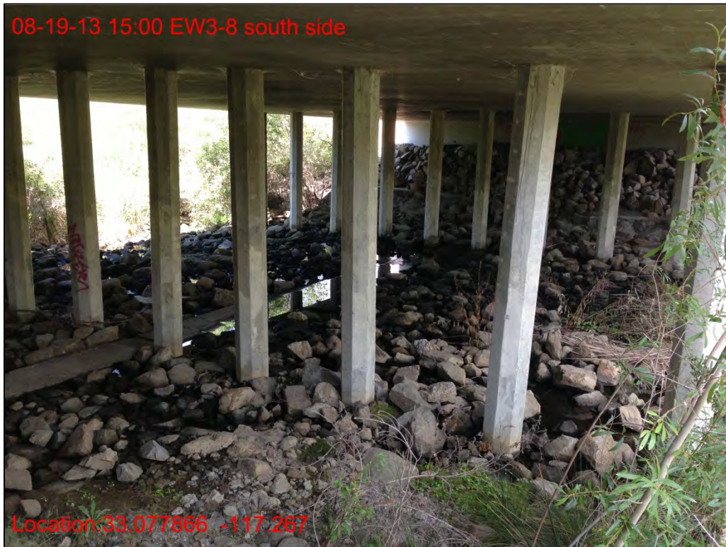
EW3-8, looking northeast from south entrance, August 2013.
