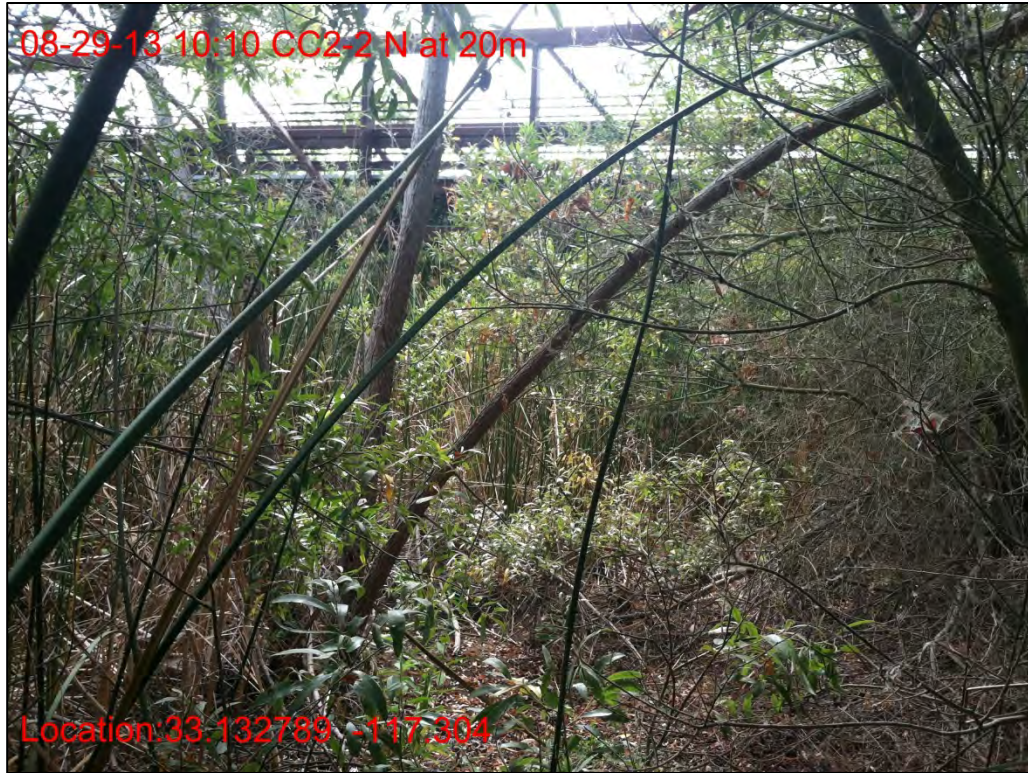
CC2-2, looking south from north side, August 2013.
