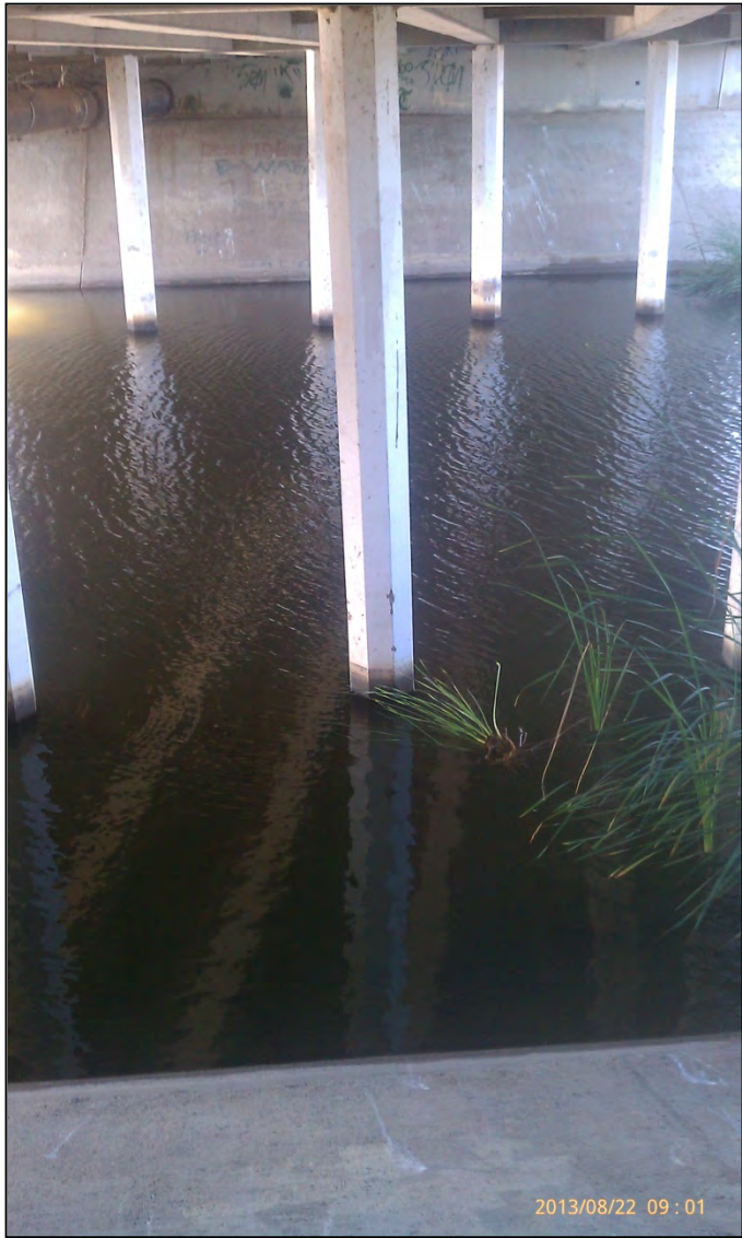
EW1-3, interior looking south from N side, August 2013.
