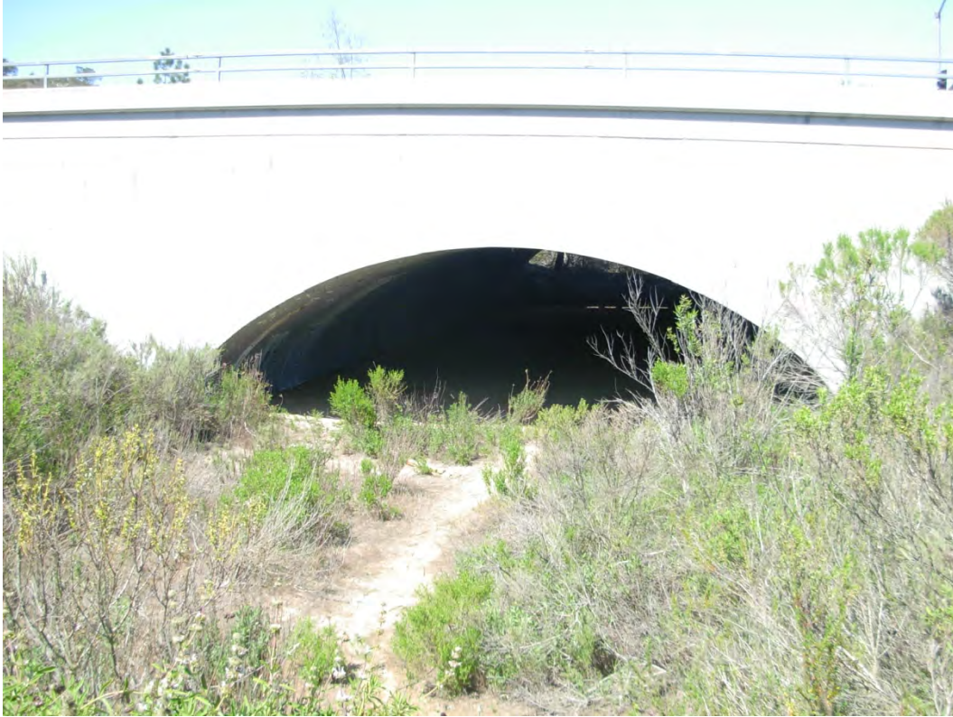
M10-1, south entrance looking north at 20 meters.
