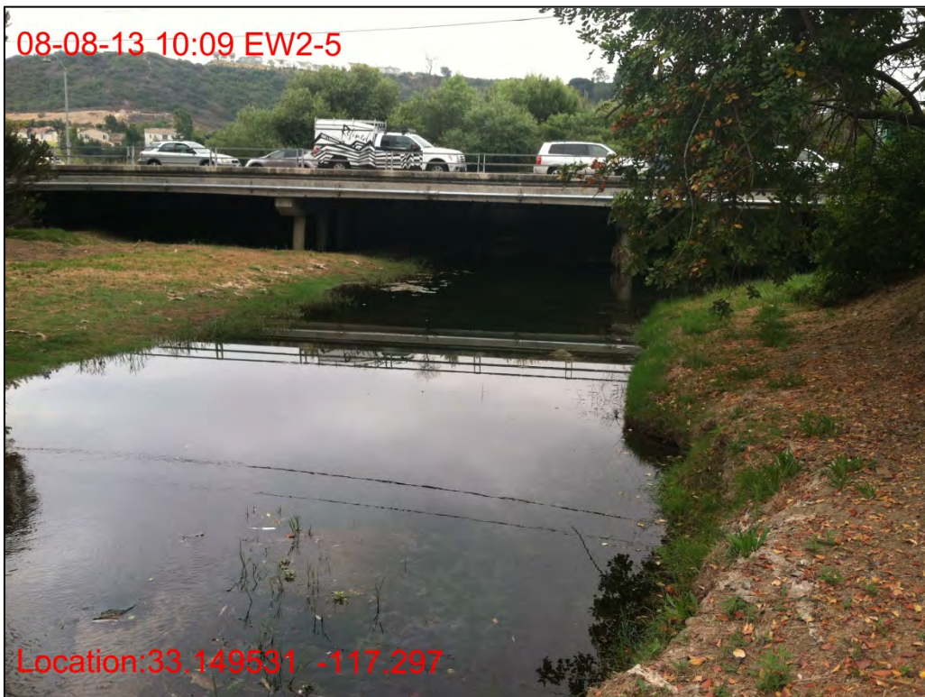
EW2-5, looking south at 20 meters from north entrance, August 2013.
