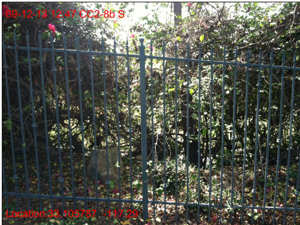
CC2-8b, fencing on south side, September 2013.
