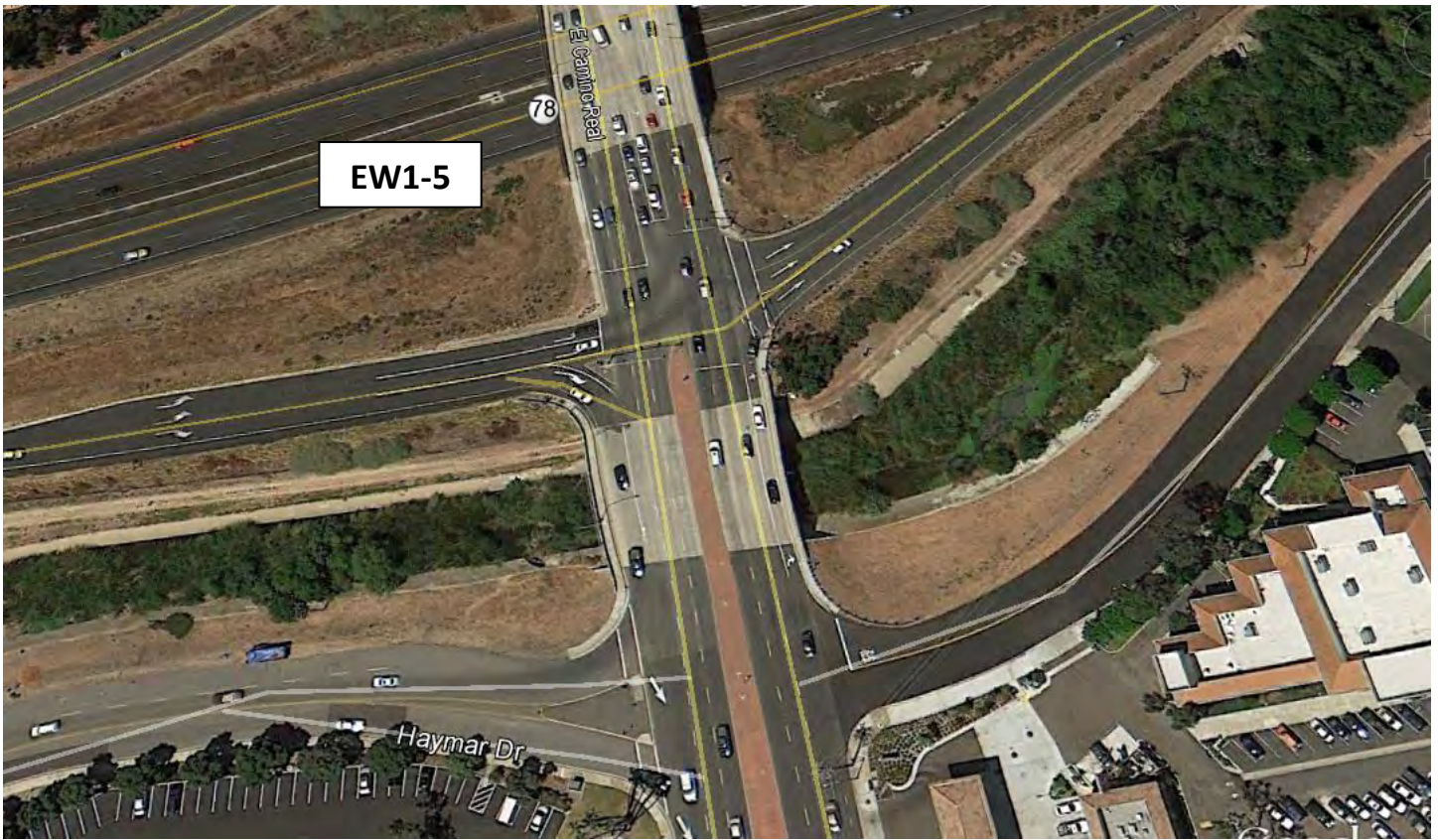
EW1-5. High Priority. Buena Vista Creek and El Camino Real. This location was recommended by the MHCP for monitoring.
