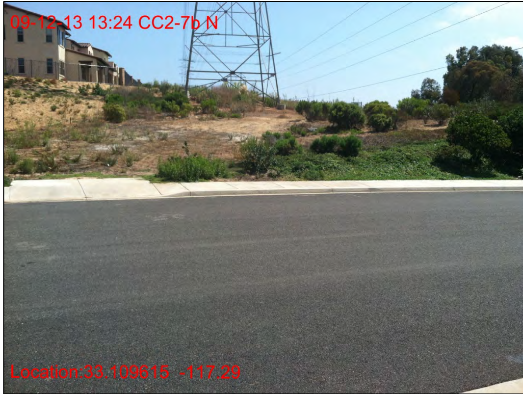
CC2-7b, at-grade crossing looking south from north side, September 2013.
