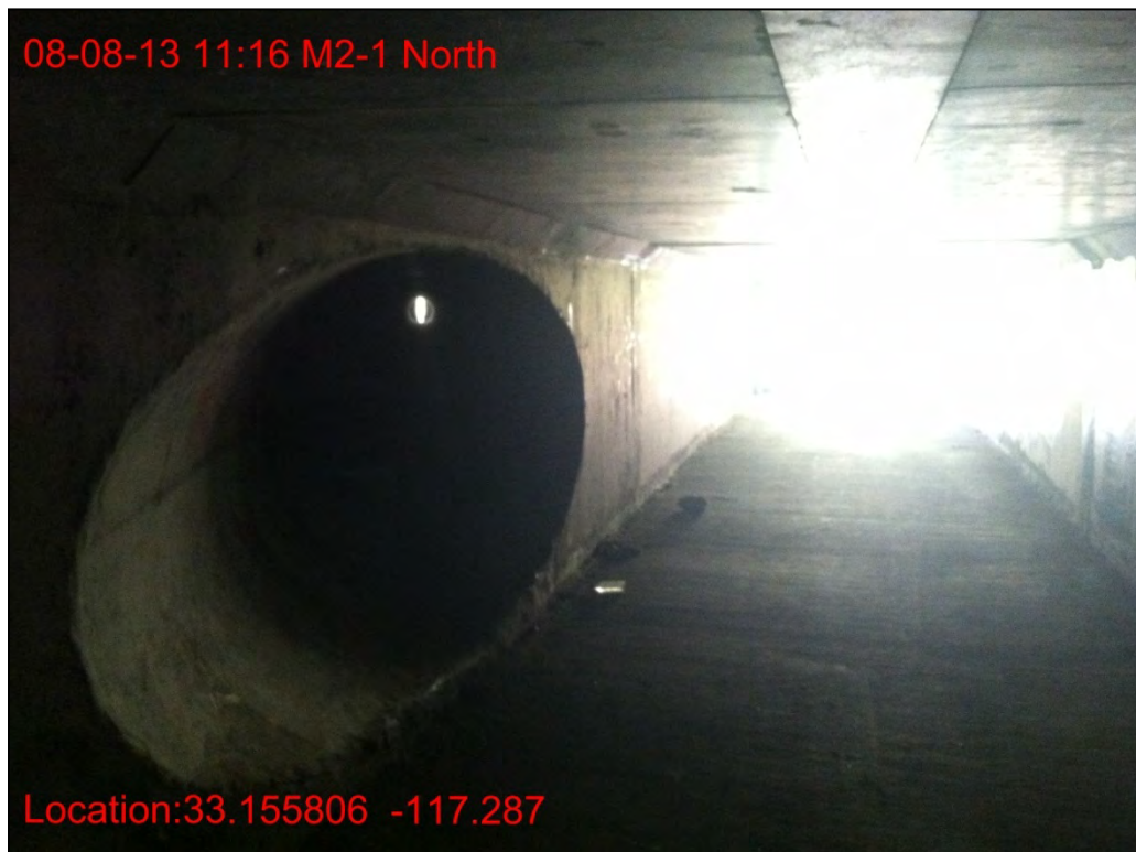
M2-1, north side facing north, showing offshoot pipe, August 2013.
