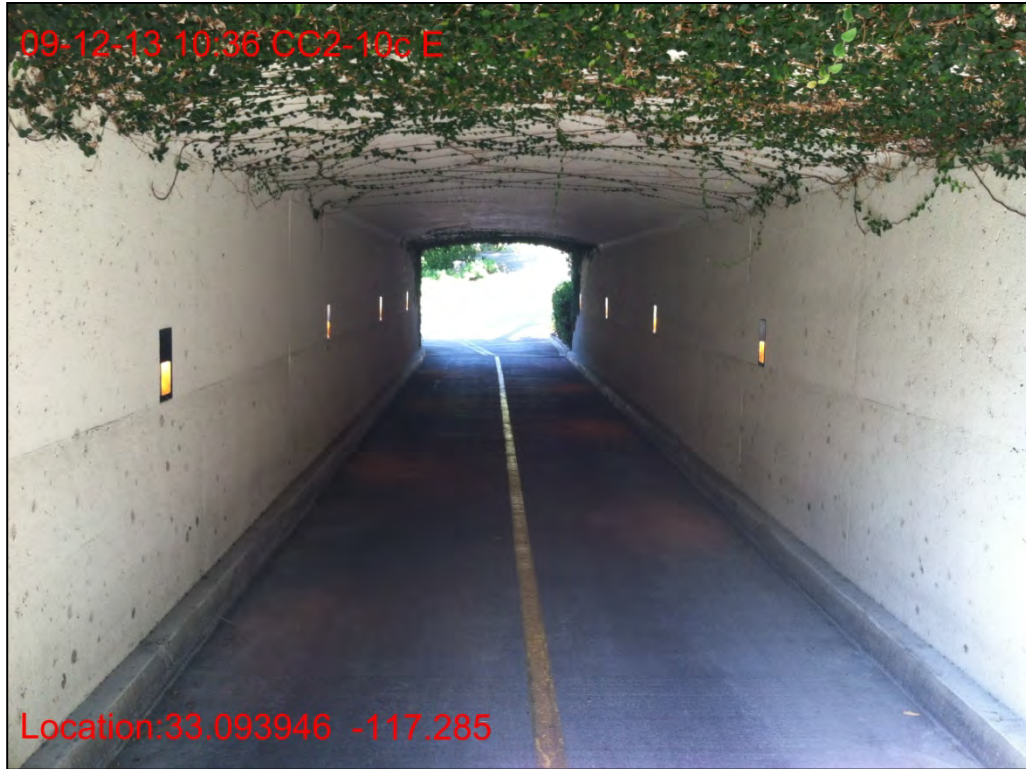
CC2-10c, east side facing undercrossing, September 2013.
