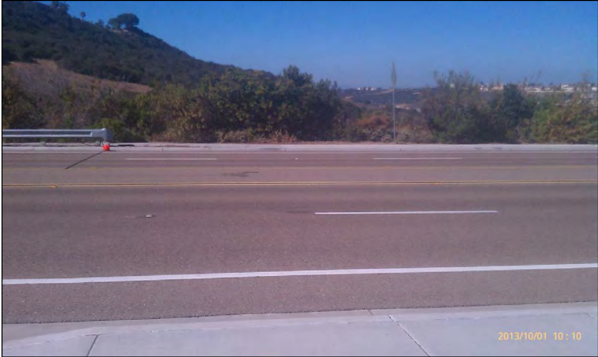
CC3-3a, at-grade crossing, east side looking west, October 2013.
