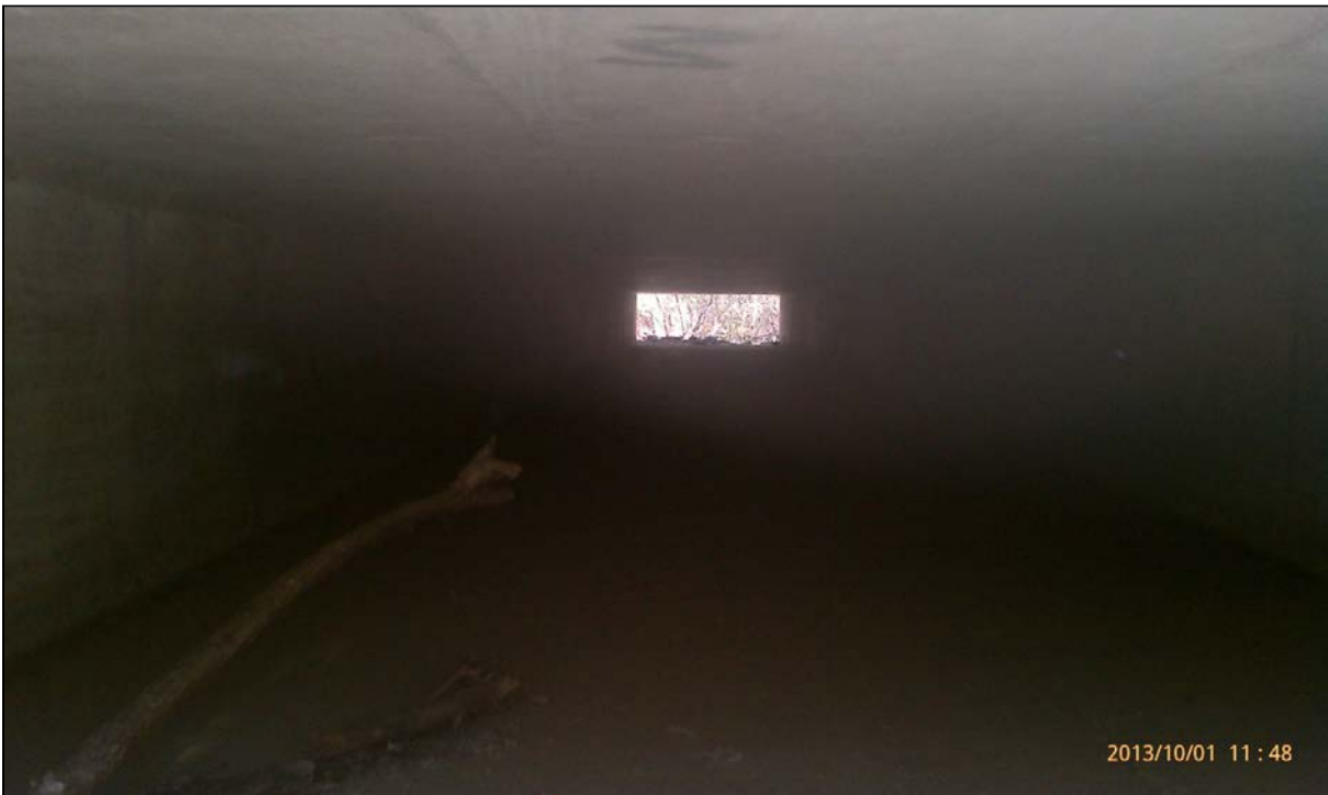
M6-3 east entrance facing toward undercrossing, showing low ceiling, October 2013.
