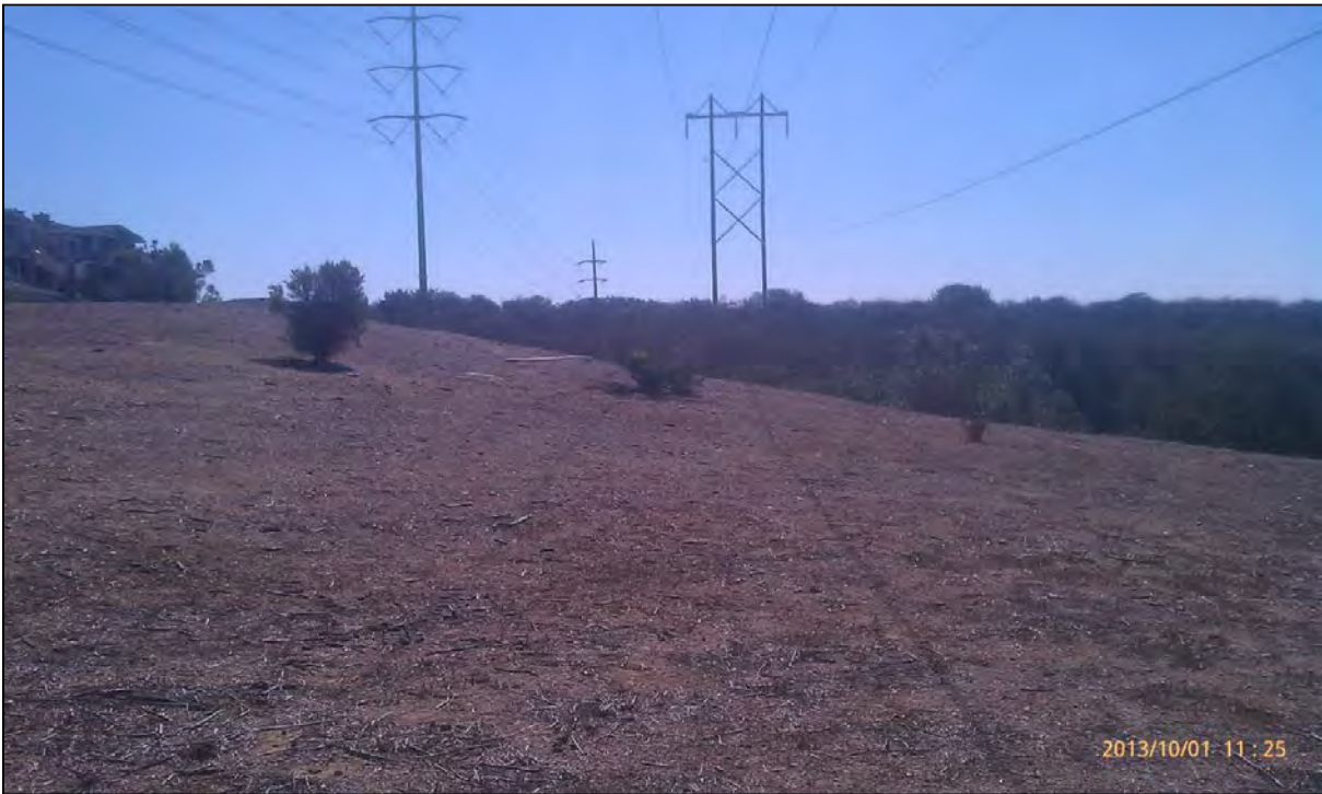
M6-4, south side facing south, October 2013.
