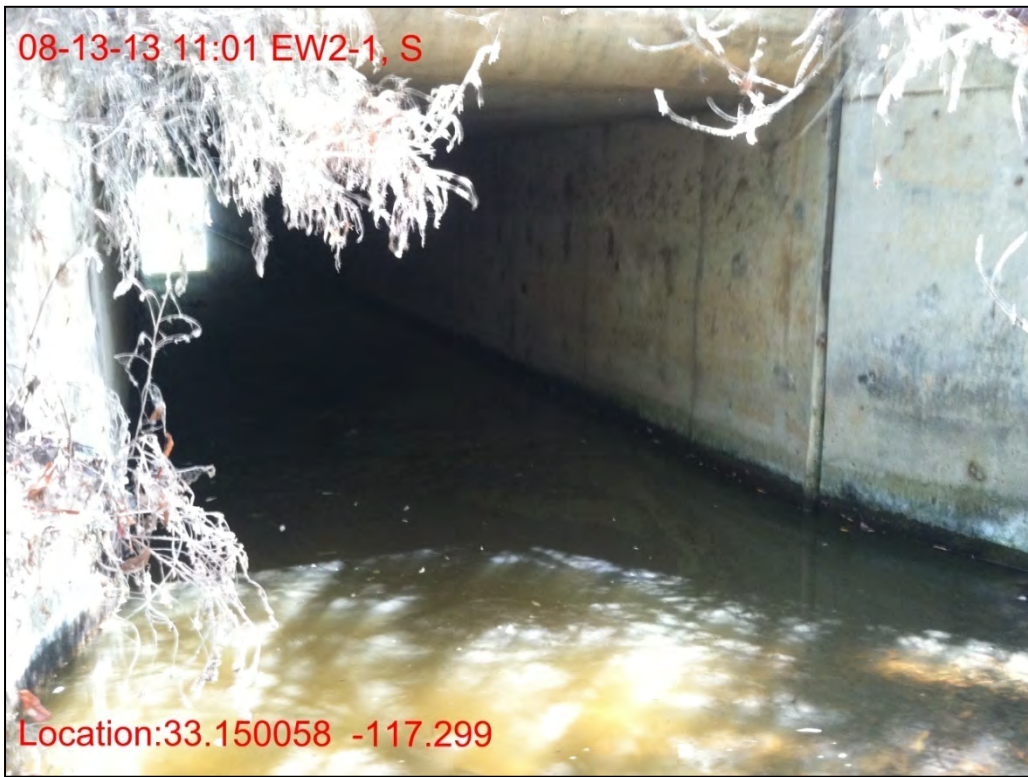
EW2-1, southern entrance showing permanent water August 2013.
