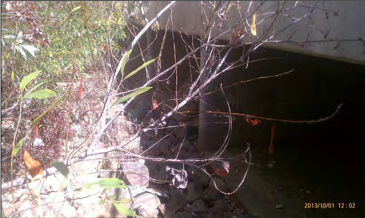
M6-1 east side looking southwest, October 2013.
