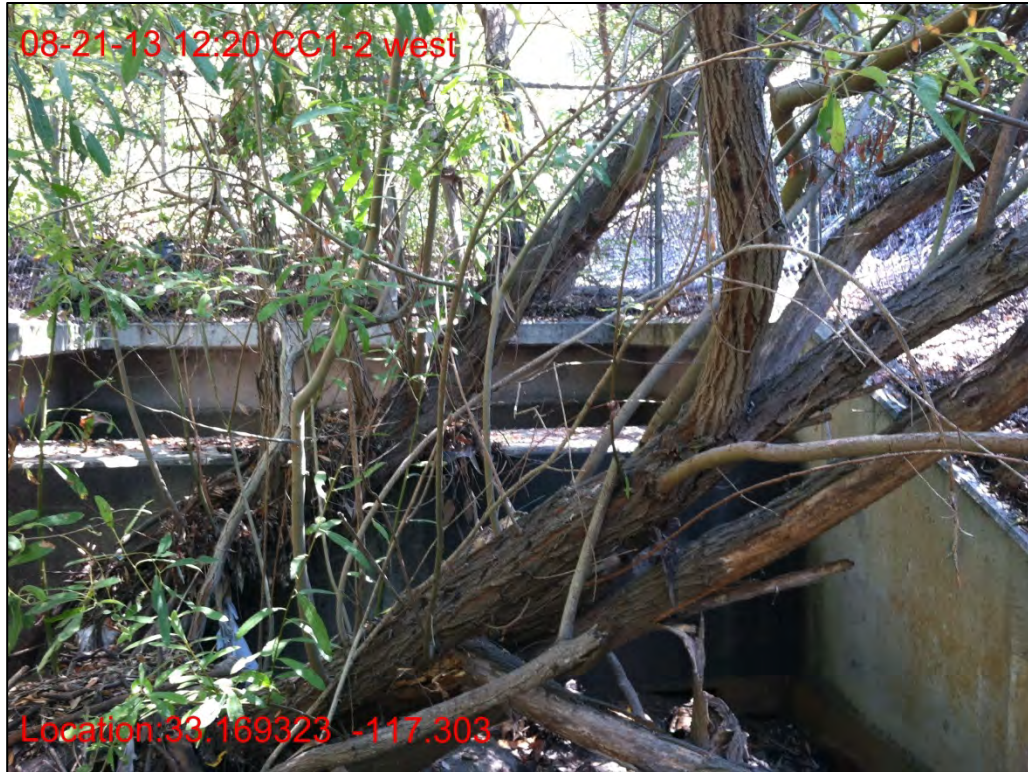
CC1-2, looking east from west side, August 2013.
