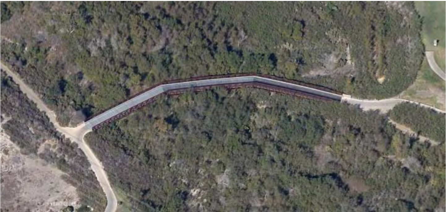
CC2-2- bridge for golf cart traffic. Not likely to be impediment to movement.
