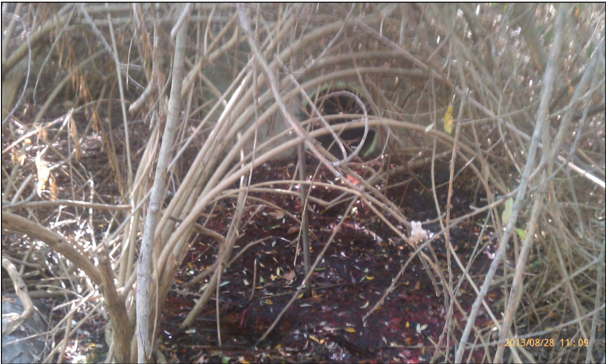
M1-1, north side showing small pipe outlet, August 2013.
