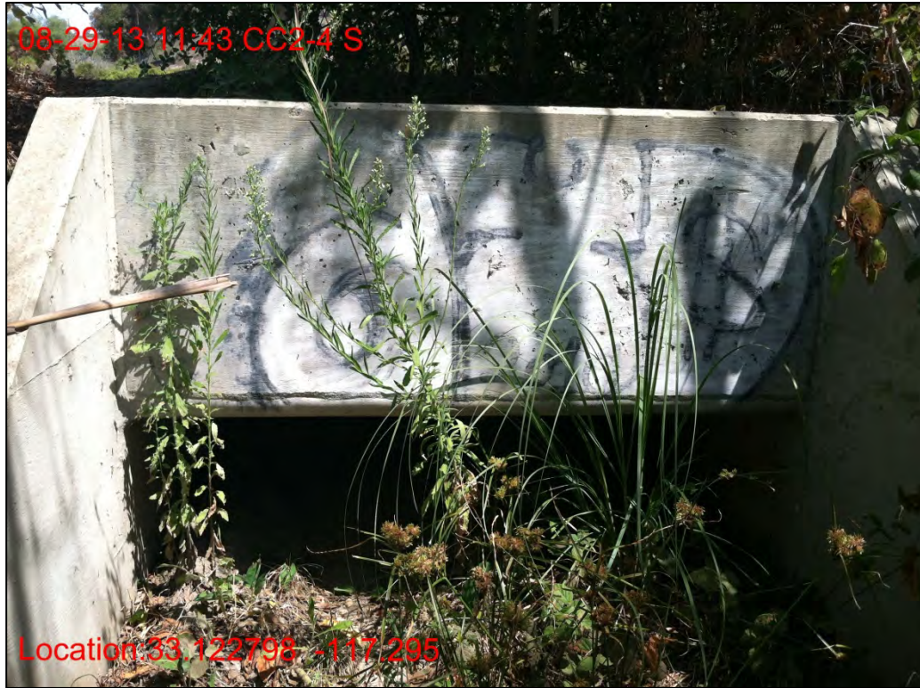
CC2-4, looking north from south entrance of culvert, August 2013.
