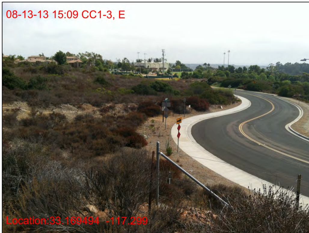
CC1-3, looking south from east side, August 2013.
