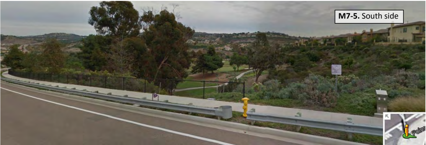
M7-5. Chain link fence along S side of Poinsettia Lane; but there is a gap on the W end, which would allow wildlife movement. Chain link fencing on N side is continuous from El Camino Real to just before Alga Norte Park.
