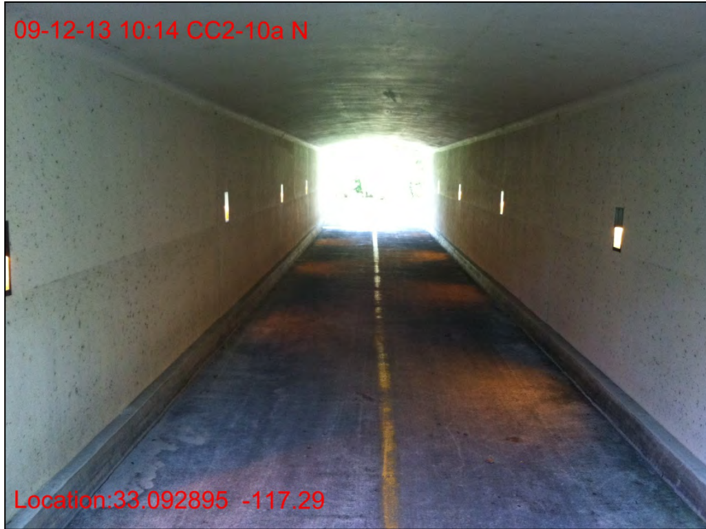
CC2-10a, north side facing into undercrossing, September 2013
