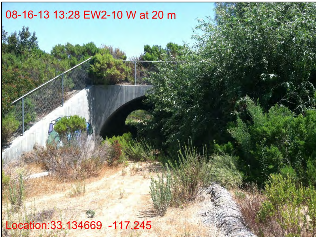
EW2-10, looking east at 20 meters from west entrance, August 2013.
