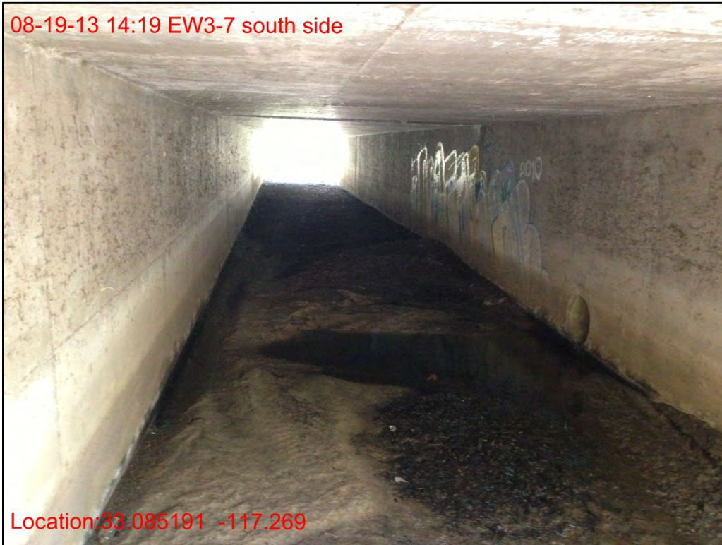
EW3-7, looking north from south entrance, August 2013.
