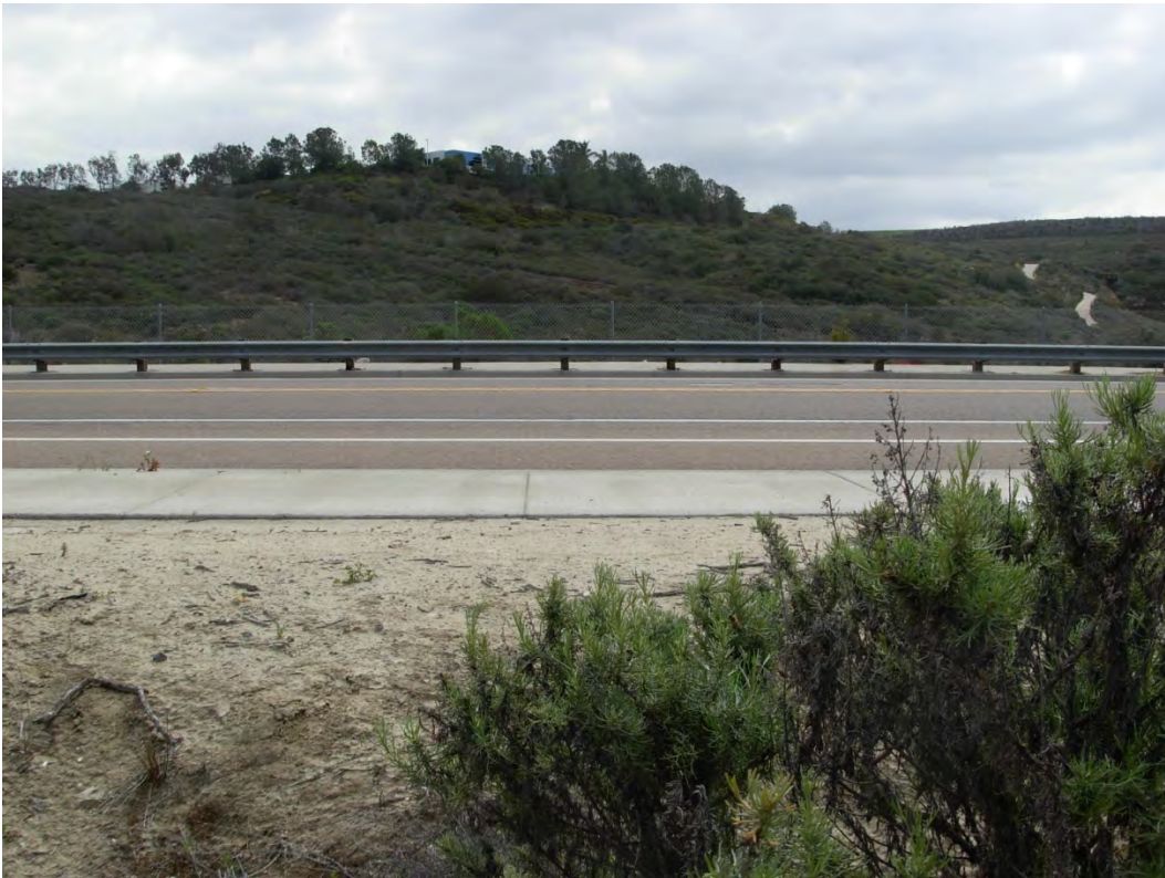
M5-2b, north side looking south.
