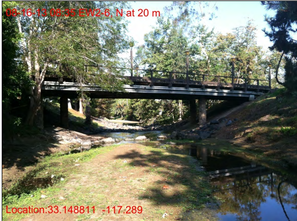
EW2-6, north side at 20 meters, August 2013
