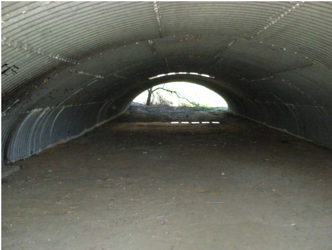
M10-1, looking north from interior.
