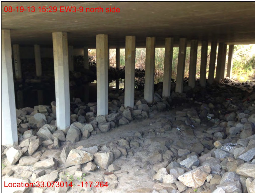
EW3-9, north side underneath, August 2013.
