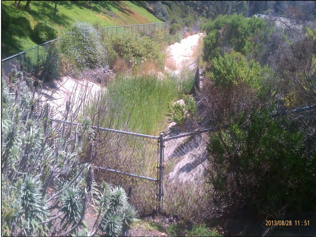
M1-4, looking north from west end, August 2013.
