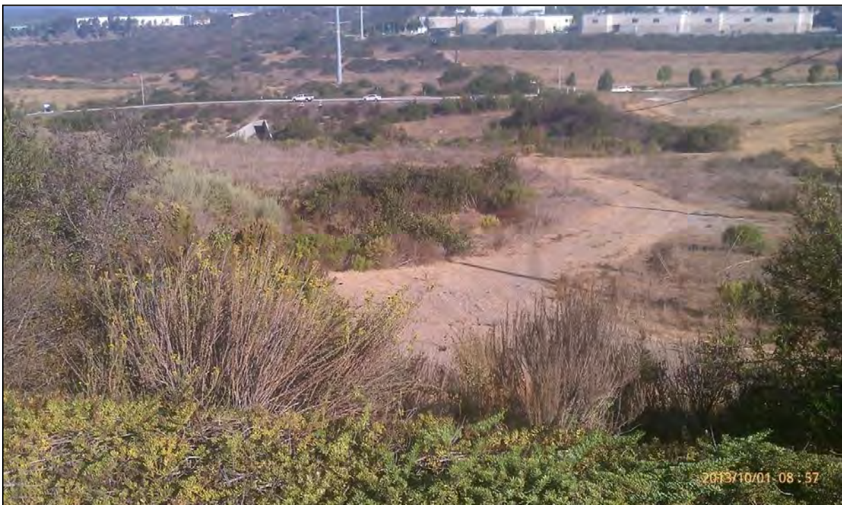
CC3-5, north side looking north (line of sight to M7-5), October 2013
