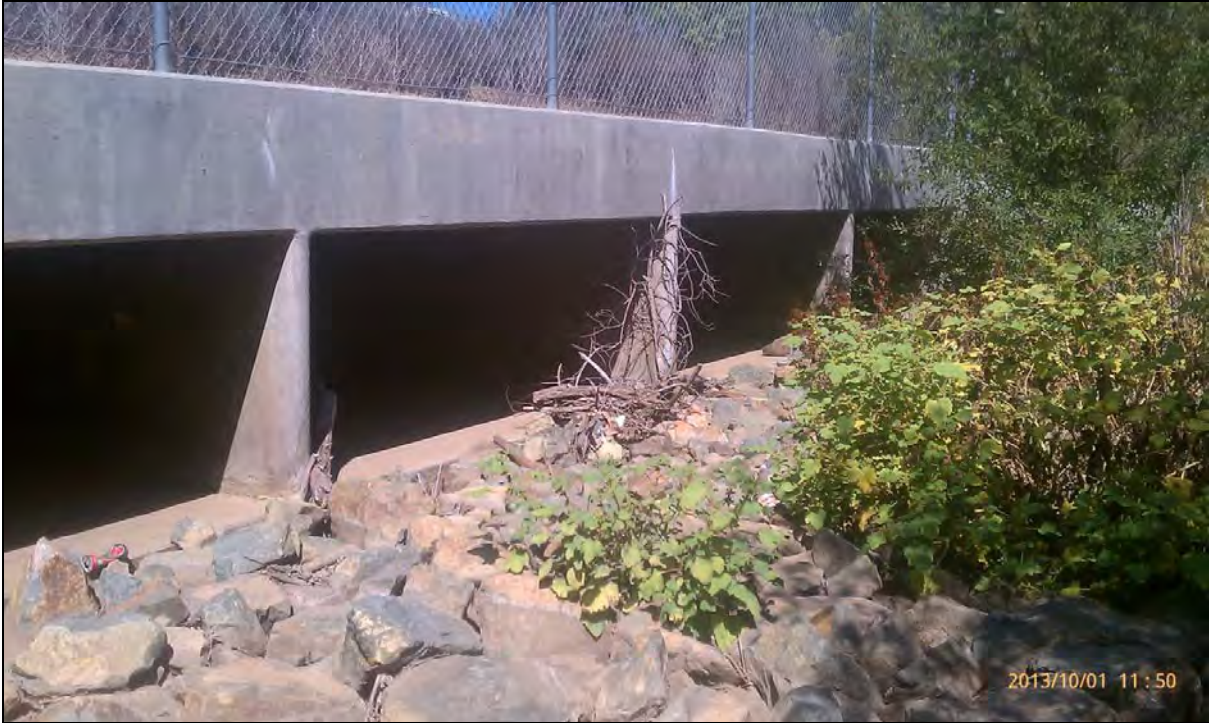
M6-3, west entrance facing southeast at multi-chambered undercrossing, October 2013.
