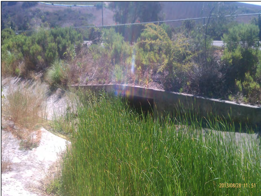
M1-4, looking east from west end, August 2013.
