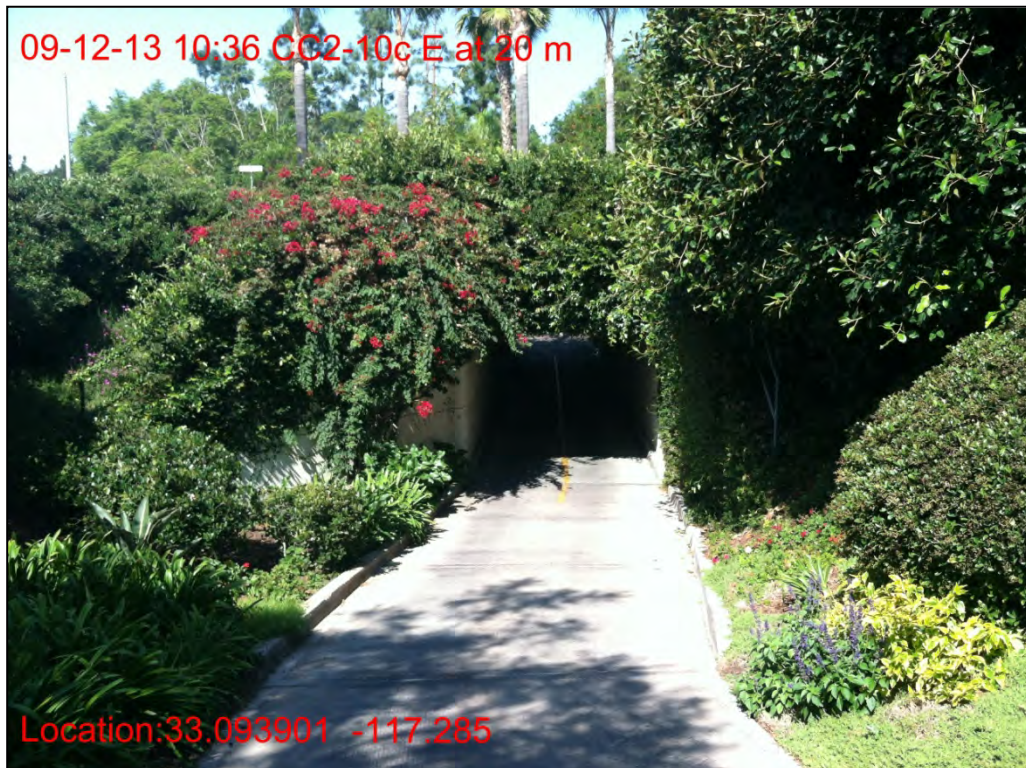
CC2-10c, east side facing undercrossing, September 2013
