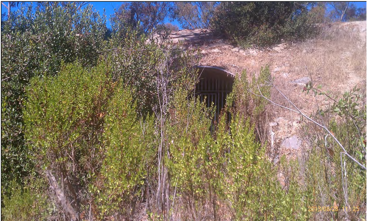
M1-2 east side facing west, August 2013.
