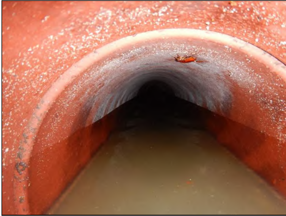
East Influent Pipe
