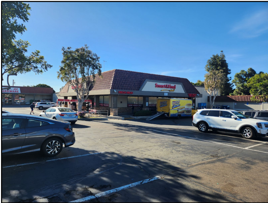
Plate 5.2–1: Overview of the project from the northwest corner of the property, facing south.
