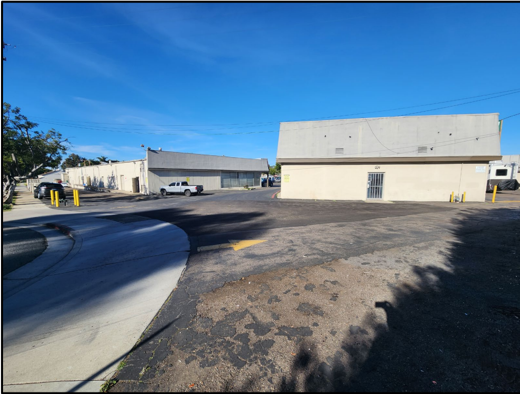
Plate 5.2–2: Overview of the project from the southwest corner, facing north.
