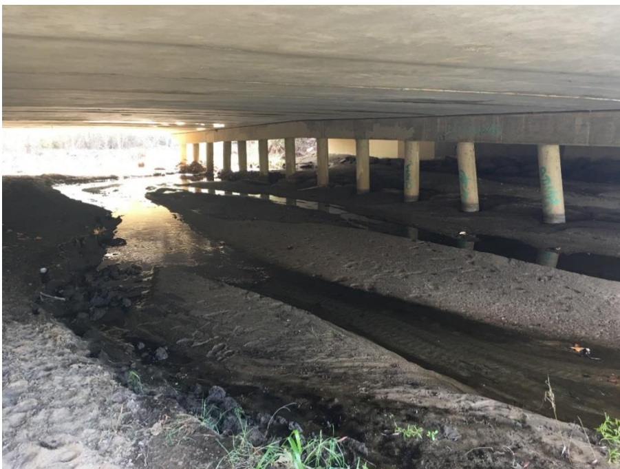
Looking south underneath the underpass at EW2-5
