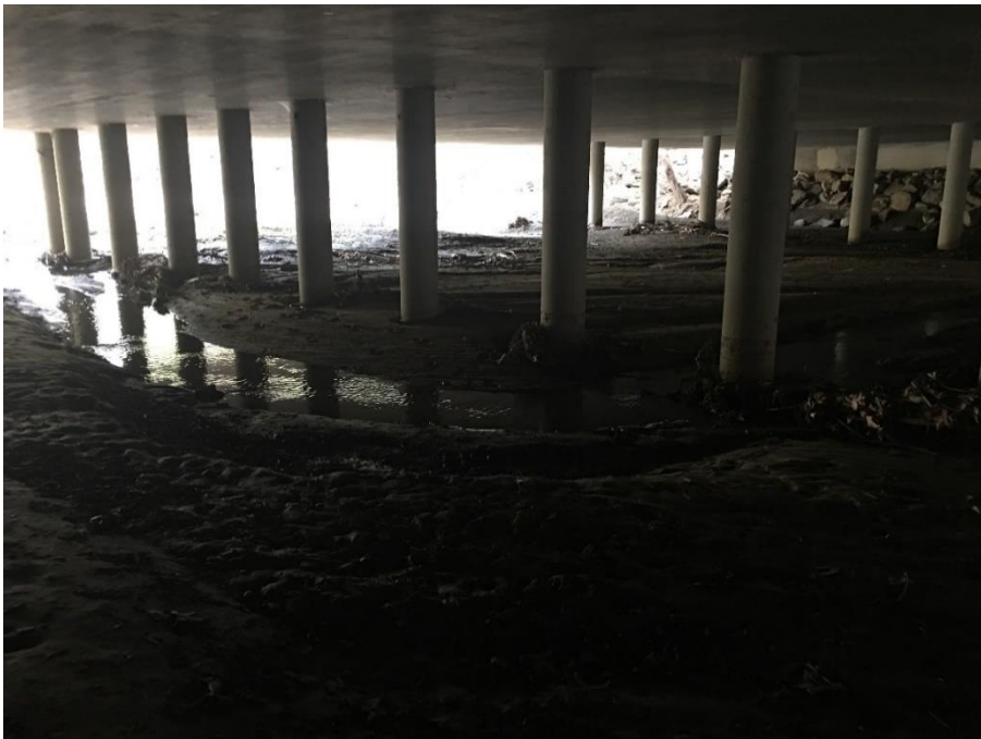
Looking east underneath the underpass at EW2-4
