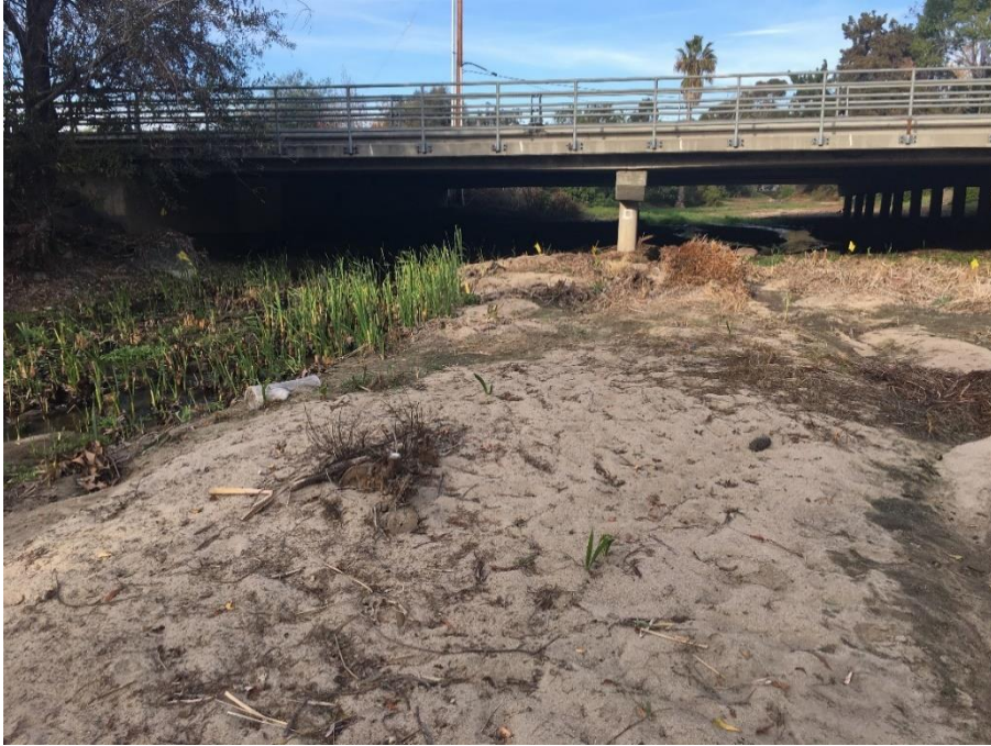
Looking northeast toward the El Camino Real underpass at EW2-5
