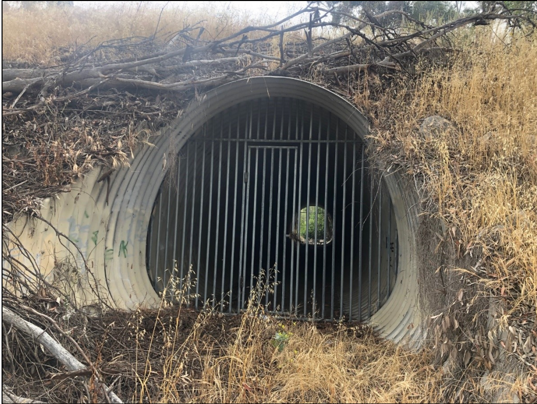
Gated culvert at M1-2 pinch point.
