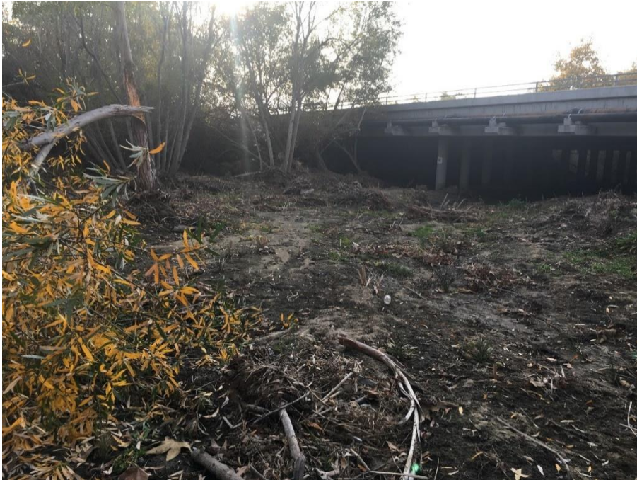
Looking southwest toward the Cannon Road underpass at EW2-4
