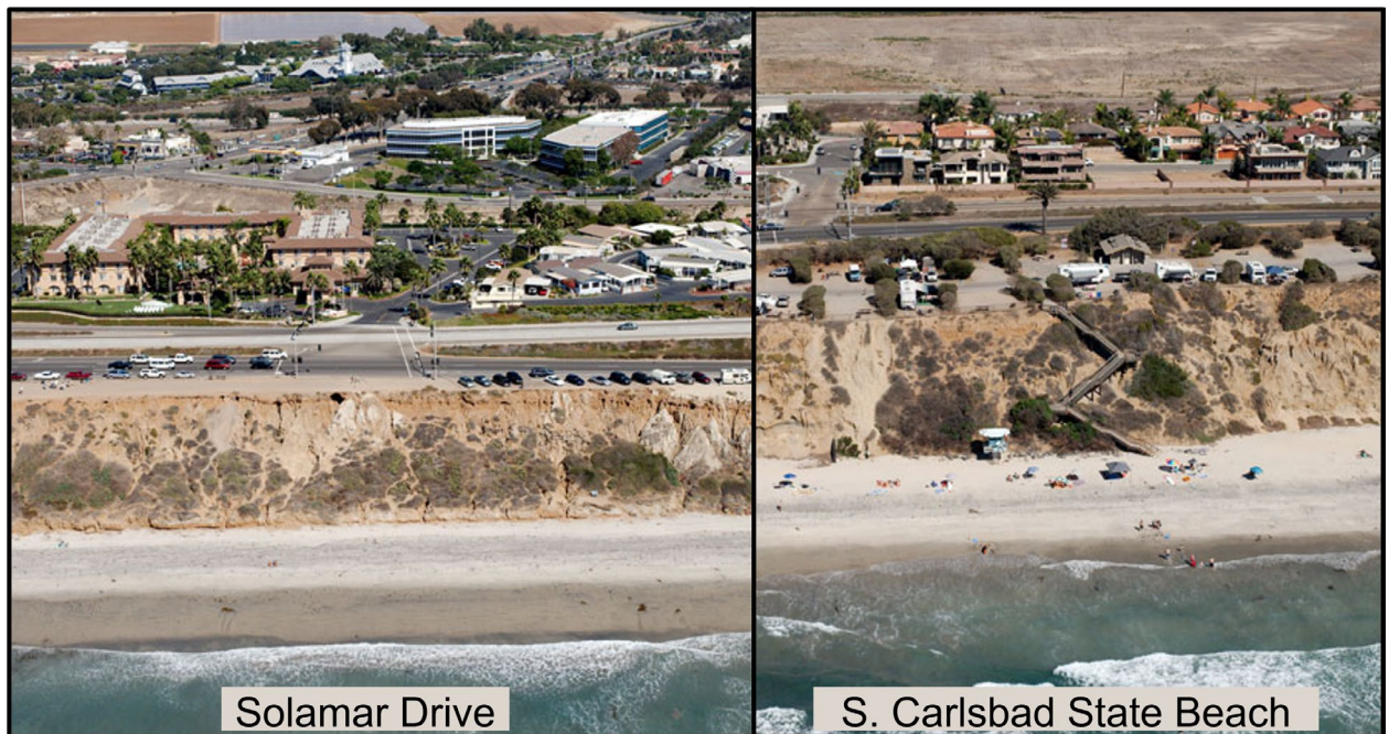
Figure 19. Current Intersection at Solamar Drive and Informal Beach Accessways (left) Compared with a Nearby Example of a Formalized Staircase at South Carlsbad State Beach (right) as an example to inform Option 2.
