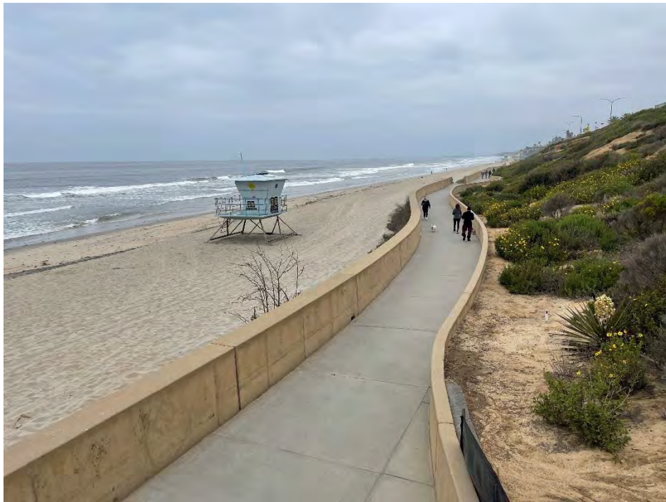
N. Carlsbad 4 (looking north from vicinity of Tower 36 stairway) – April 25, 2023
