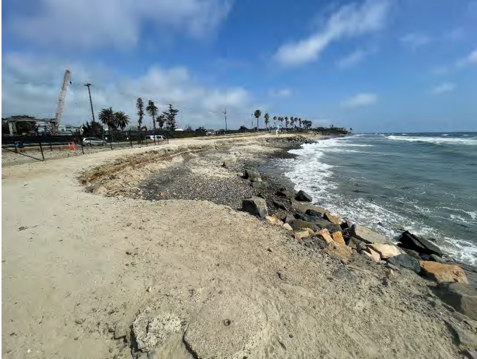
S. Carlsbad 1 (looking south from Agua Hedionda Outlet South Jetty) – April 25, 2023
