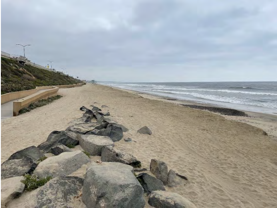
N. Carlsbad 1 (looking south from north end of seawall) – April 25, 2023
