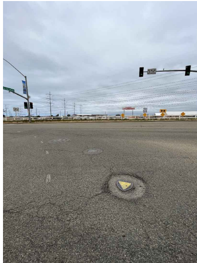
PHOTO 1 - FROM SOUTH LOOKING NORTH
