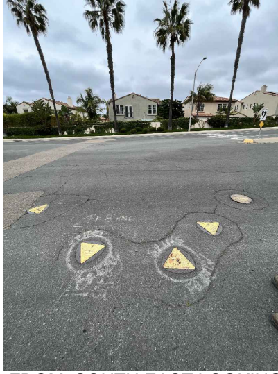
PHOTO 1 - FROM SOUTH EAST LOOKING NORTH WEST
