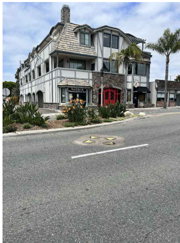
PHOTO 1 - FROM SOUTH EAST LOOKING NORTH WEST
