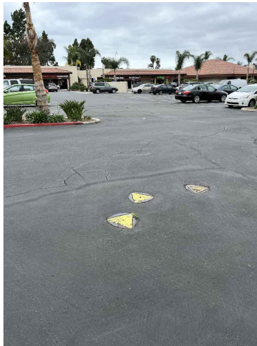
PHOTO 1 - FROM EAST LOOKING WEST
