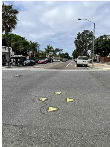
PHOTO 1 - FROM SOUTH EAST LOOKING NORTH WEST ON ROOSEVELT ST
