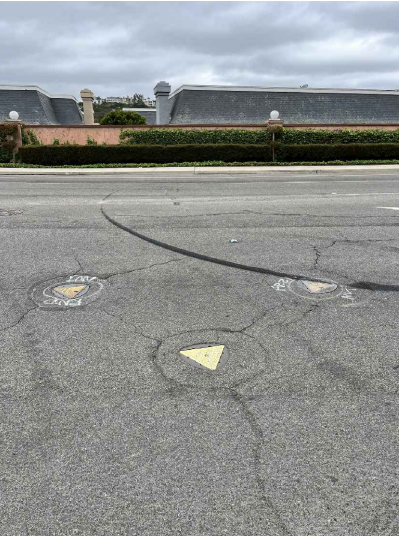
PHOTO 1 - FROM NORTH LOOKING SOUTH
