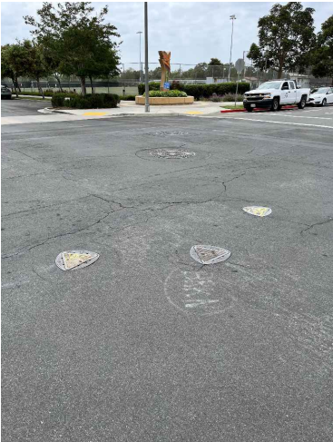
PHOTO 1 - FROM EAST LOOKING WEST
