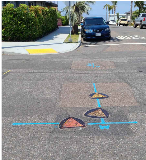
PHOTO 1 - FROM SOUTH EAST LOOKING NORTH WEST ON GARFIELD ST
