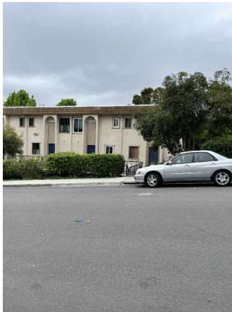
PHOTO 1 - FROM SOUTH LOOKING NORTH AT 2352 ALTISMA WAY
