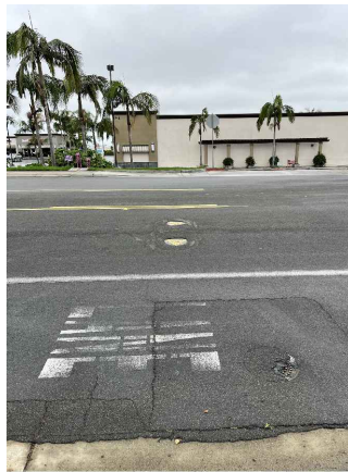
PHOTO 1 - FROM EAST LOOKING WEST
