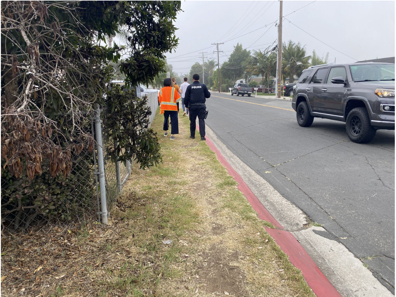
Missing sidewalk on the east side of Jefferson Street between Tamarack Avenue and Chinquapin Avenue.
