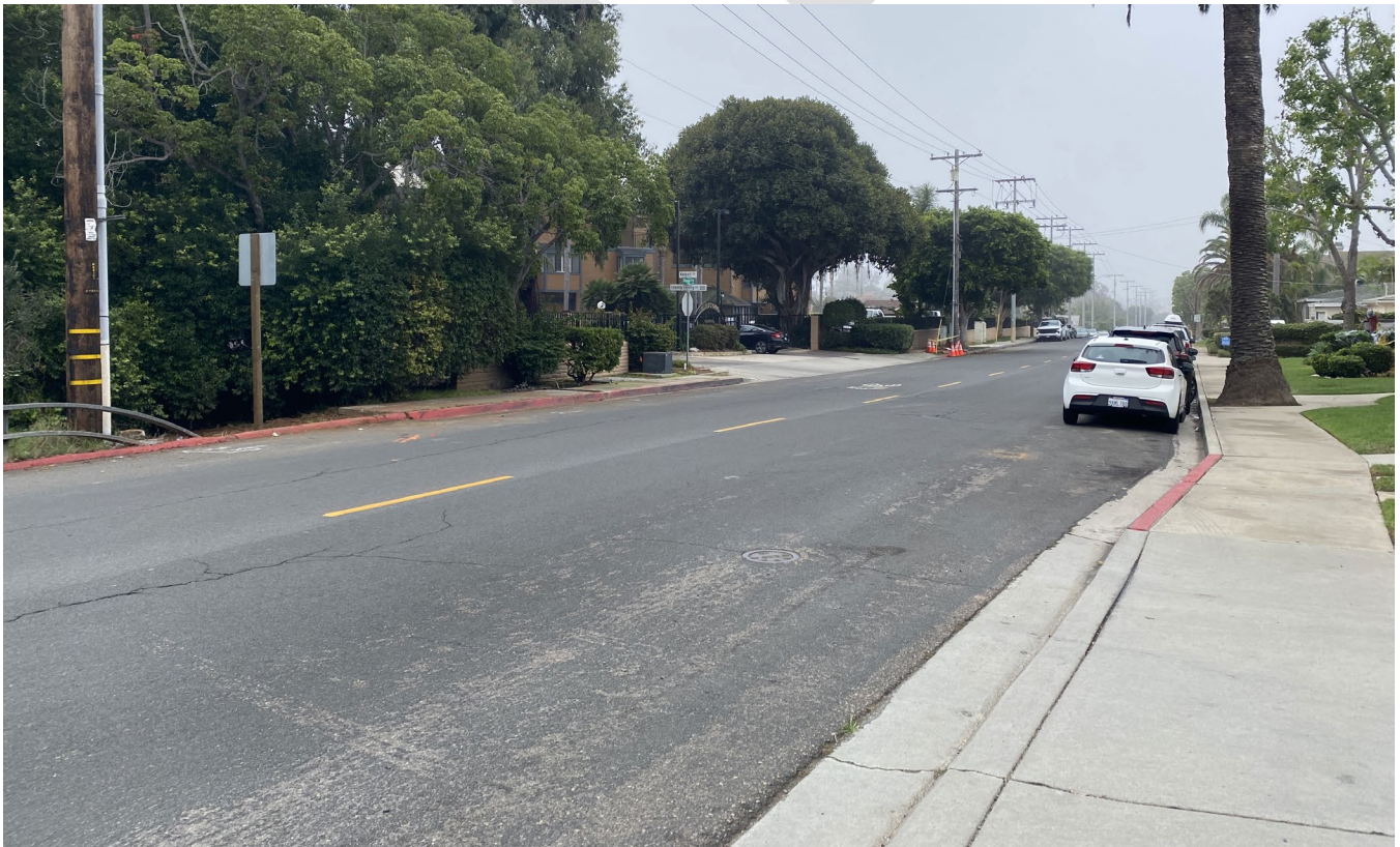
Narrow and inconsistent sidewalk on both sides of Chinquapin Avenue.
