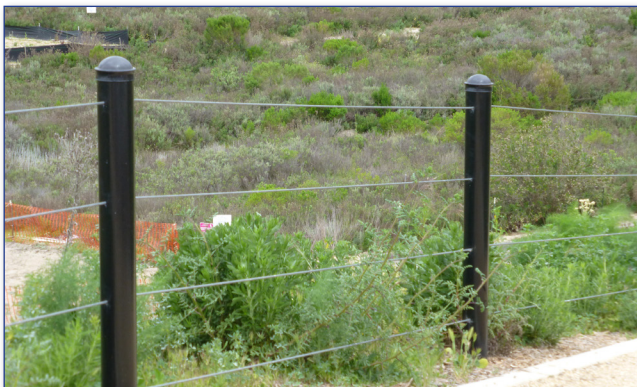
Metal post and cable
