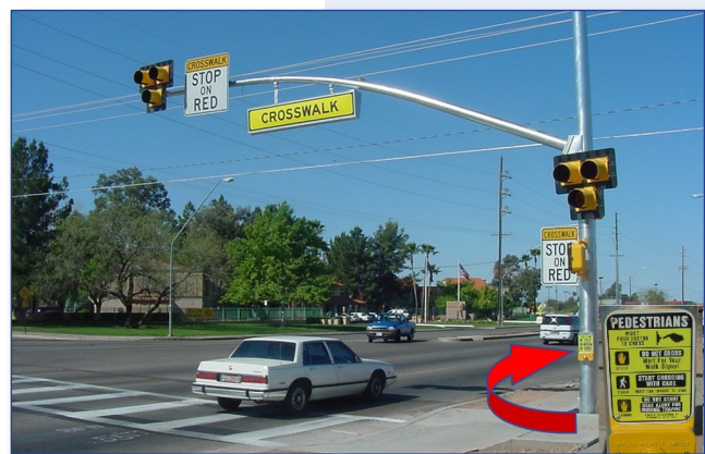
Multiple lanes require positive protection such as this Rectangular Rapid Flashing Beacon
