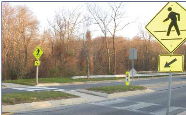
Uncontrolled crosswalks should include signage, a median refuge and a state yield law sign
