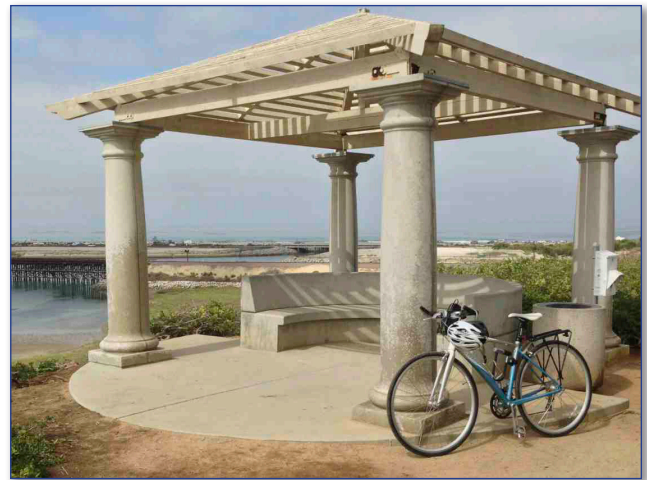
High level shade structure and benching
