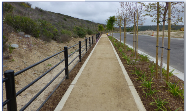
Metal post and three metal rails
