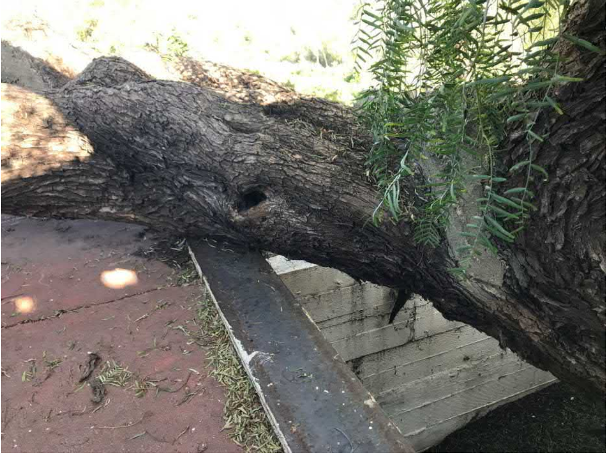
Finished installation, foam trimmed and painted with the branch resting on the steel support plate. 2018
