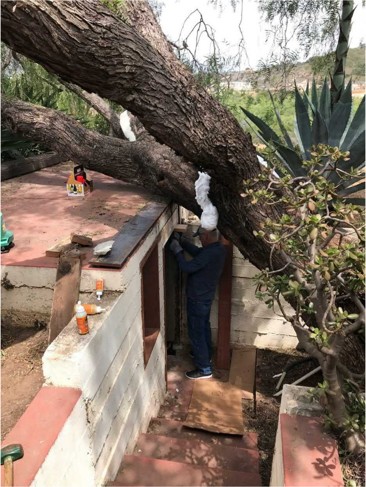
White expanding foam before trimming to conform to the shape of the branches. 2018.
