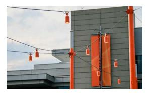
Figure 87 – Catenary Cable-mounted Lighting example with color as primary feature, daytime (D Street Corridor, Boston, MA)
