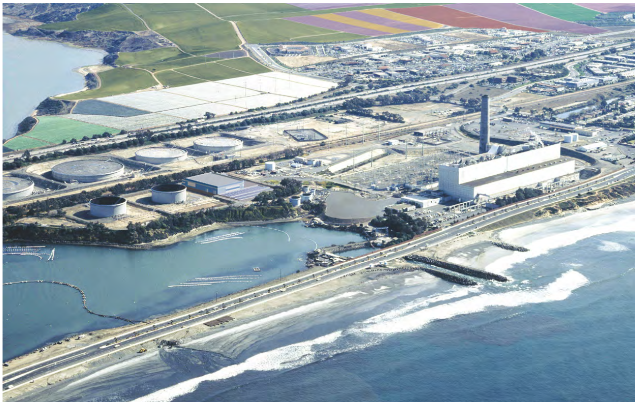
Carlsbad Power Plant and site of the Carlsbad Desalination Plant.
