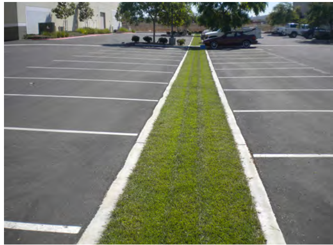
Example of green design feature: parking lot designed to drain into a natural turf area that filters and treats pollutants with organic materials.
