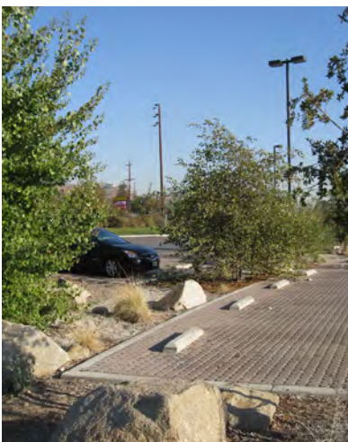
Example of water use reduction: artificial turf on athletic fields (top); example of water loss reduction: parking lot with porous paving (bottom).
