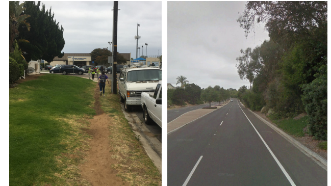
Missing Sidewalks in Carlsbad; residential area (left) and high-speed roadway (right)
