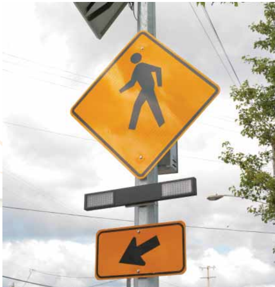
Rectangular Rapid Flashing Beacon (RRFB) Device Portland, Oregon
