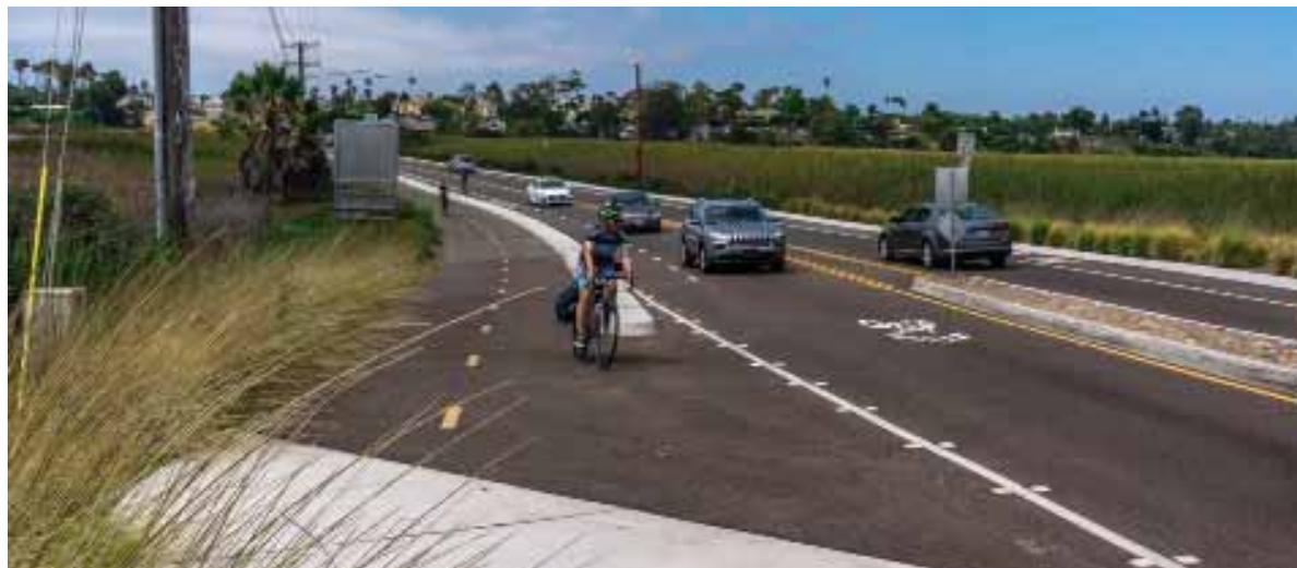
Bicycle Facility Transition – Carlsbad
