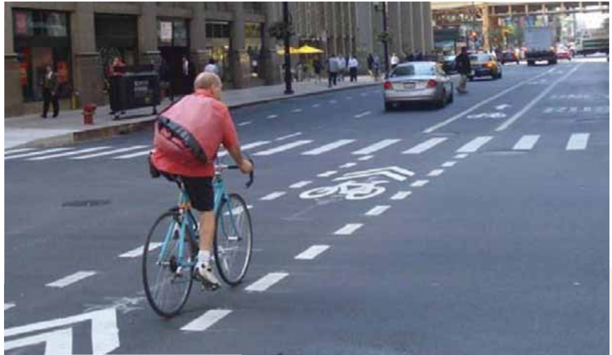
Bicycle Intersection Treatment – Minneapolis, Minnesota
