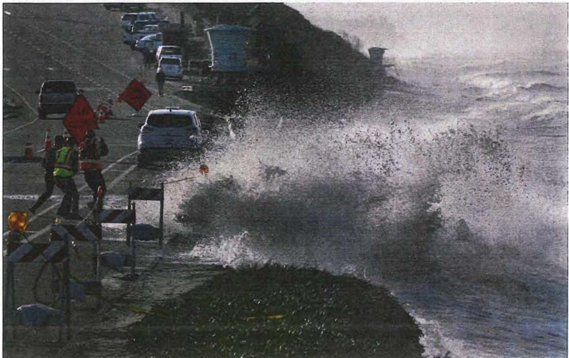
Photo 8. Erosion and Flooding at Las Encinas Bridge
