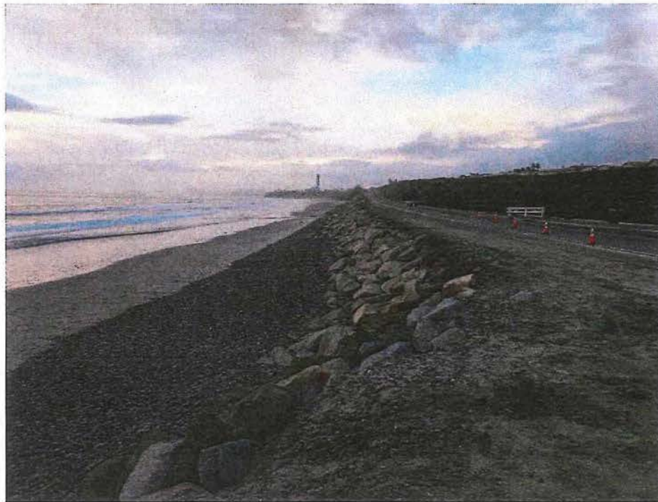
Photo 6. Existing Revetment at Las Encinas Bridge
