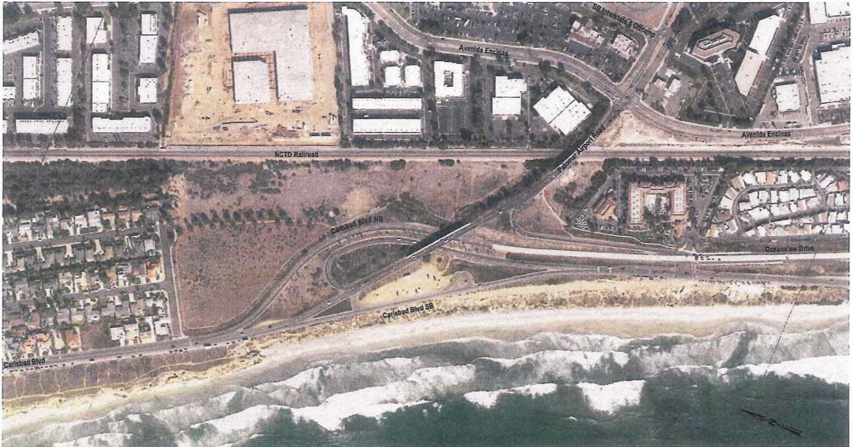
Attachment 1b: Map showing Carlsbad Boulevard split between Northbound and Southbound lanes and proximity to bluff and beach
