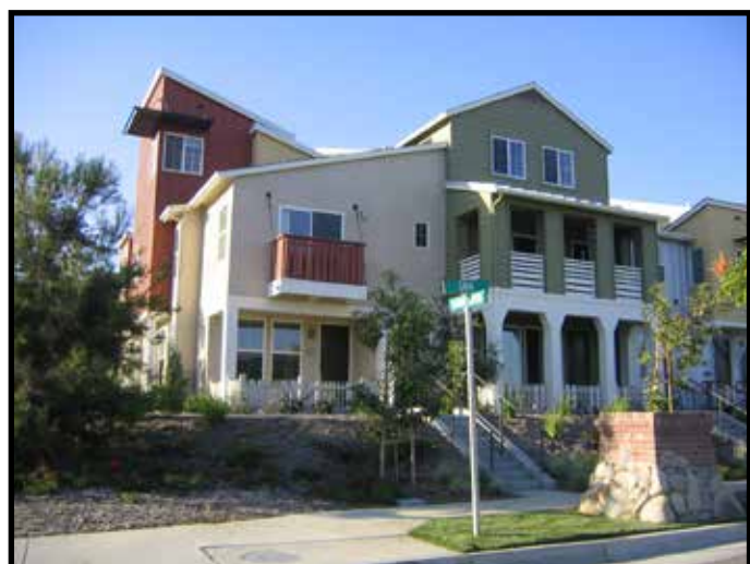
Articulated roof forms
