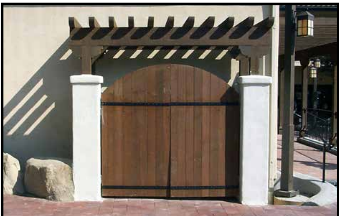
Screened service area
