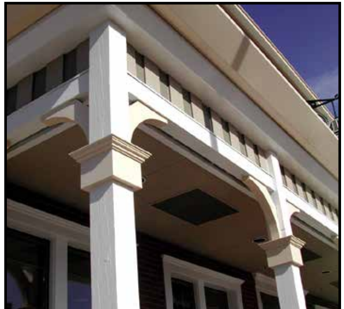
Appropriately sized and functional column
