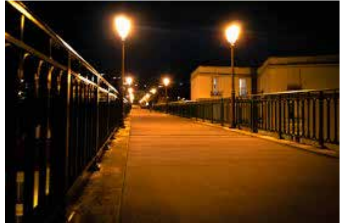
Night street lighting
