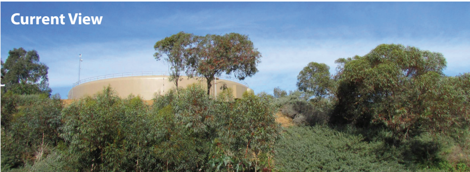
View with New Tank
