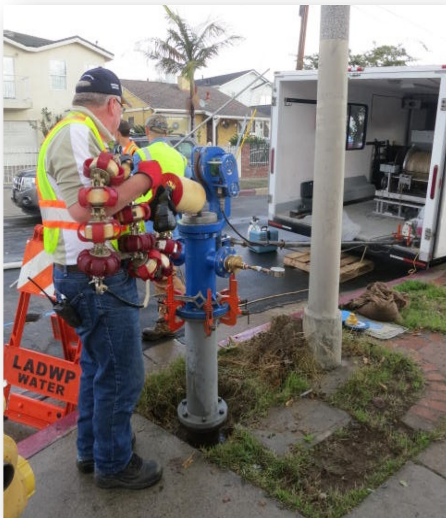
Figure 3-23. Example of Small Diameter In-Pipe Electromagnetic Technology
