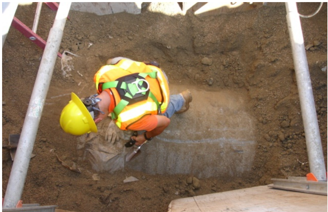
Figure 3-21. Example of Targeted Excavation and Measurement of Pipe Wall Thickness
