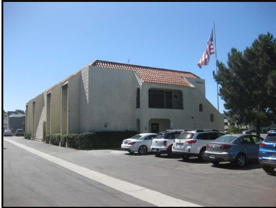
View of the building on the subject property, facing south.
