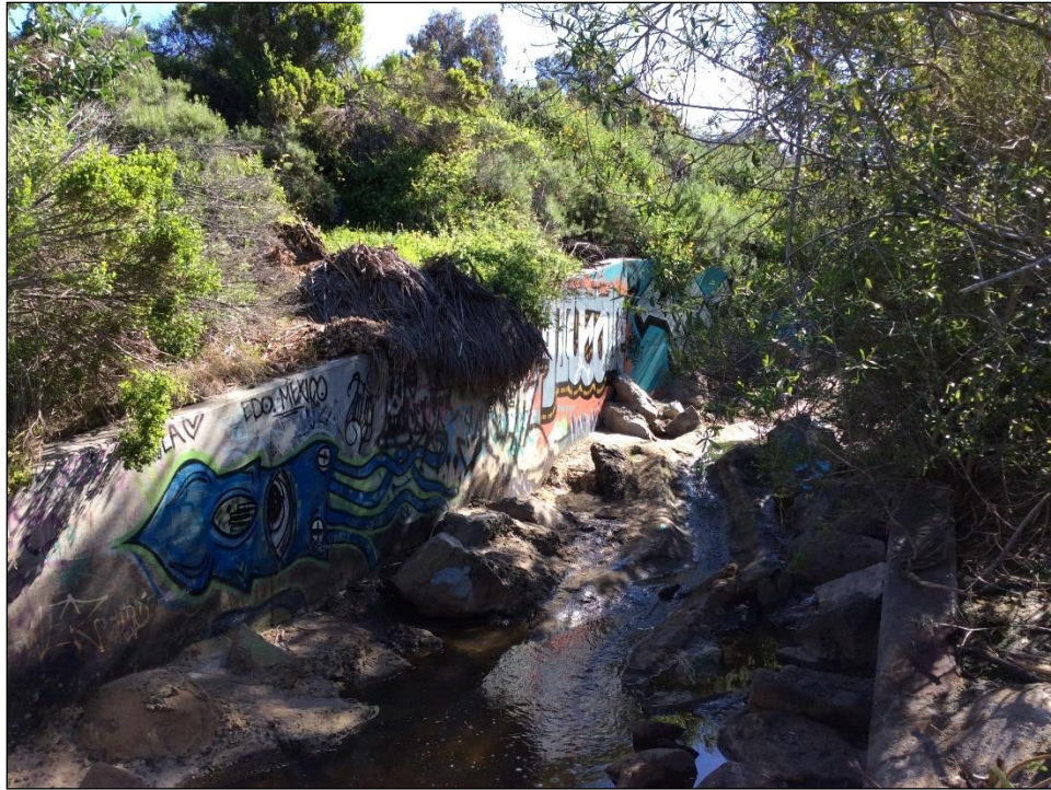
Figure 5 Cemented cobbles within drainage channel, view facing southeast.
