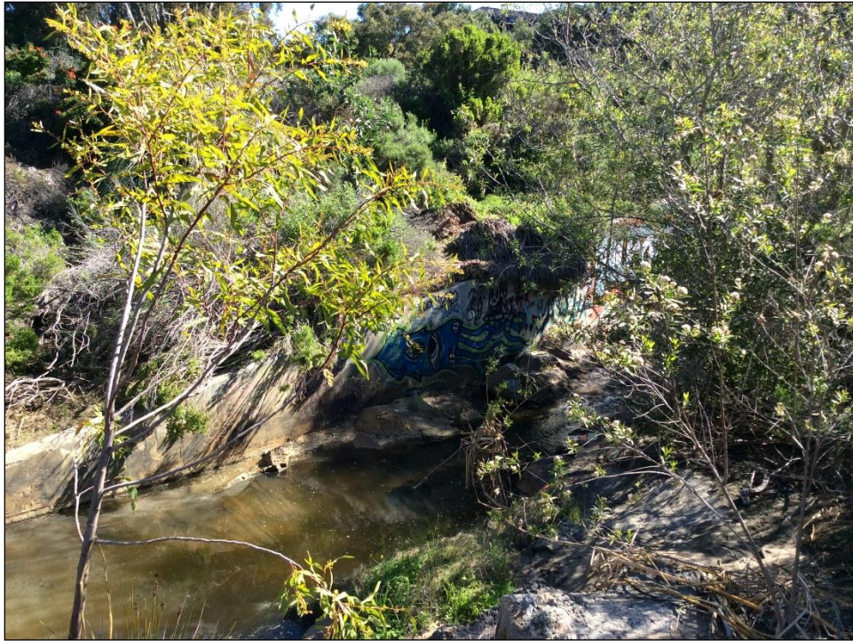
Figure 3 Drainage Channel in northern portion of project area, view facing southeast.
